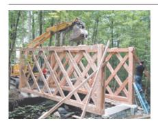
3. The completed trusses were eased into position with an excavator and supported by temporary braces while the bridge deck and roof structure were added. The far end of the span is supported by an outcropping of ledge leveled with a little concrete, and the near end by a concrete-block wall faced with stone from the site. The ends of the trusses rest on 4x12 slabs of rot-resistant white oak.
