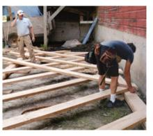
1. After laying each truss member in place, Kellogg bored three or four holes at each crossing point and fastened the assembly with kiln-dried ash pegs. The pegs swelled on contact with the green lumber, holding it solidly in place.
