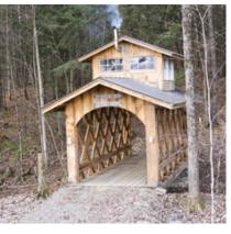
**4.** The almost-finished bridge (the bottom half of the trusses will eventually be protected by board siding) is as sturdy and useful as it is handsome. Kellogg reports that it easily bears the weight of a tractor carrying a load of firewood from his woodlot to the house.
