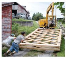
2. Strapped to a couple of hardwood skids, the first truss was dragged a half-mile to the bridge site — a laborious operation that was not repeated. The second truss was built on the banks of the stream, with juice for the power tools provided by a generator.
