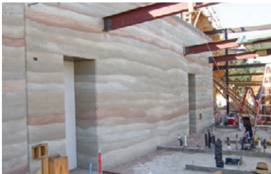
Mineral soils were trucked from several quarries to achieve the desired color coordination. Embedded steel columns support the adjoining floors and roofs.
