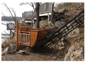
Among the lift's safety features are an interlock gate system that prevents the car from moving unless closed and latched, and an automatic braking system that engages if the car speed exceeds normal limit or slack is detected in the cable.
