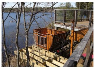
The four-passenger car on this elevator overlooking Ontario's Muldrew Lake has been custom-finished with red cedar siding. To prevent it from blocking the view from the deck, a programmable controller sends it out of sight down the slope 15 minutes after it comes to a stop at the top station. Entering a use code on the post-mounted control panel (at right in photo) calls it back for another trip.
