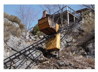
The car moves along the rails at a stately 60 feet per minute. The rectangular structure just beneath it contains the gear-driven winch and 2-hp electric motor that controls the car's motion by means of a 5/16 aircraft cable.
