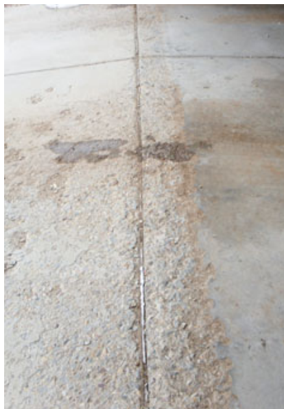
This surface spalling could have been prevented if the concrete mix had included air-entrainment.
