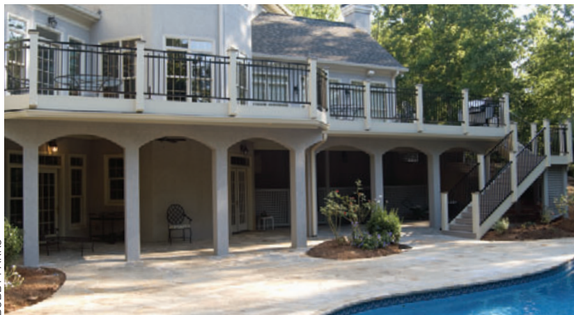
Figure 5. Building a patio below an upper deck that incorporates a drainage system gives the customer outdoor entertainment options in inclement weather.
