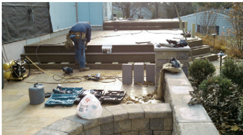
Figure 7. Some parts of the job, such as building stairs, require close coordination between the deck builder and the hardscape contractor.
