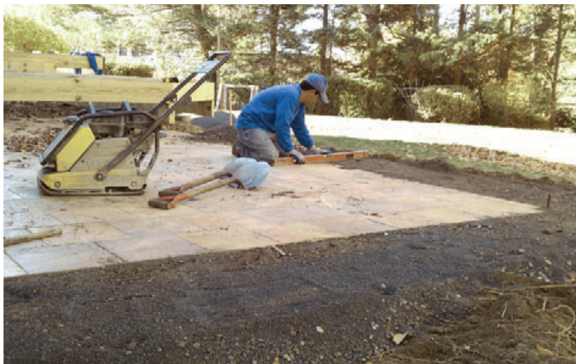
Figure 1. Patios made from concrete pavers can add space to a backyard project at a fraction of the cost of a deck.
