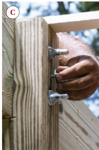
Figure 1. ThruLok screw bolts (A) provide a quick way to assemble built-up girders. They self-tap, like many wood screws (B), and are secured on the back with a wing nut (C).
