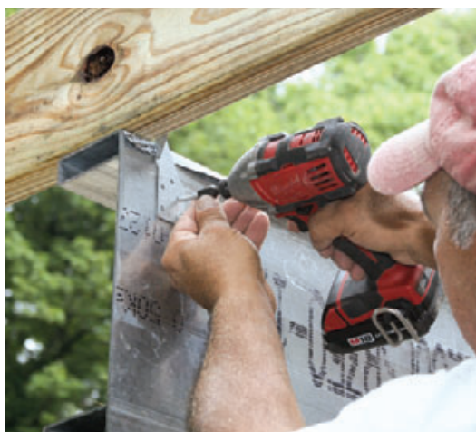
Figure 7. Carpenters set the joists for a freestanding deck (above); the band will remain spaced away from the brick veneer wall. Where joists cross the LiteSteel beam, self-tapping metal screws secure the metal ties (left). Note the strip of flashing membrane separating the pressure-treated lumber from the steel.
