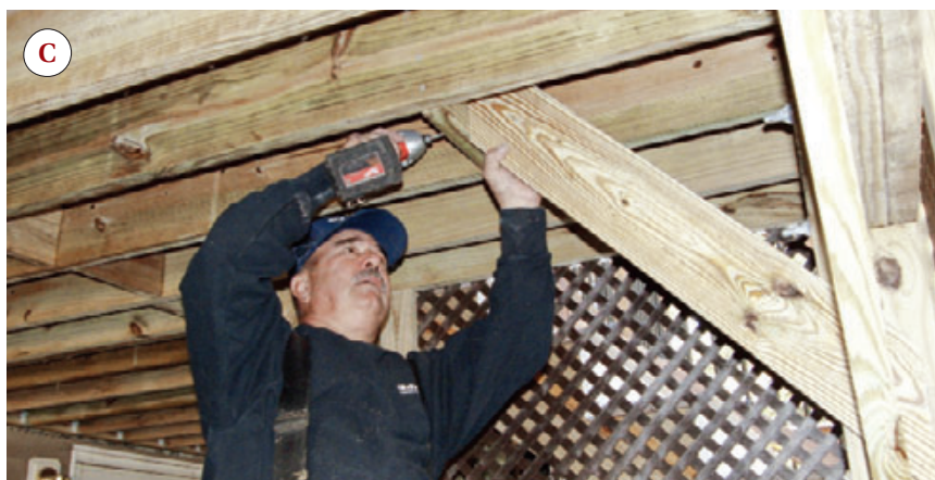
Figure 3. The author's crew installs Y-bracing (A) to resist side-to-side movement parallel to the house. Lateral braces resist movement away from the house; these are installed from each post to the side of a joist (B) or to a block between joists (C).
