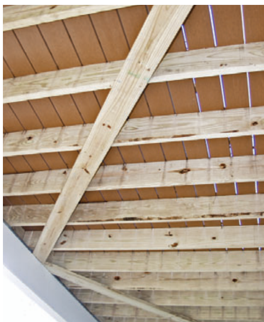
Figure 4. Whenever the decking is installed perpendicular to the joists instead of diagonally, the author uses 2x6 V-bracing to resist racking. The V-braces are attached to each joist with two screws. V-bracing is also used with many brands of grooved composite decking, which is typically installed with clips that do not resist horizontal forces.
