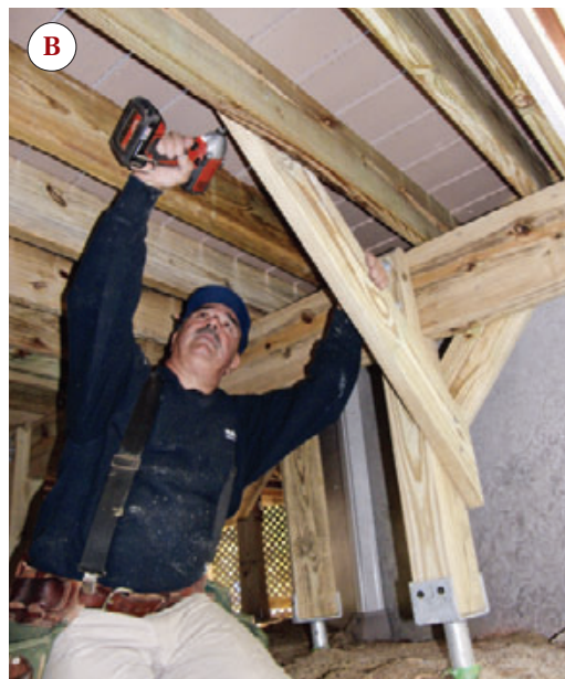
Figure 3. The author's crew installs Y-bracing (A) to resist side-to-side movement parallel to the house. Lateral braces resist movement away from the house; these are installed from each post to the side of a joist (B) or to a block between joists (C).
