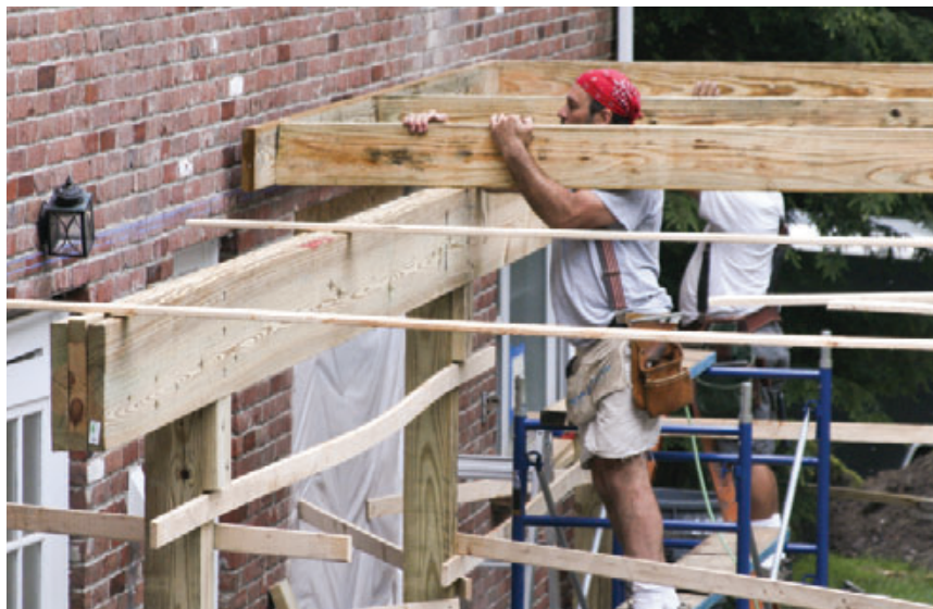
Figure 7. Carpenters set the joists for a freestanding deck (above); the band will remain spaced away from the brick veneer wall. Where joists cross the LiteSteel beam, self-tapping metal screws secure the metal ties (left). Note the strip of flashing membrane separating the pressure-treated lumber from the steel.
