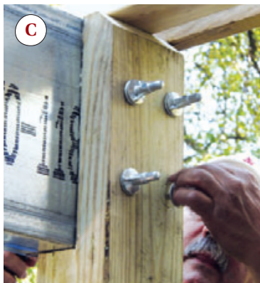
Figure 6. Using a LiteSteel beam enabled the author to eliminate a view-obstructing post in this deck project (A). Two-by-squash blocks (B), secured with ThruLok bolts (C), cinched the connection to the notched post.
