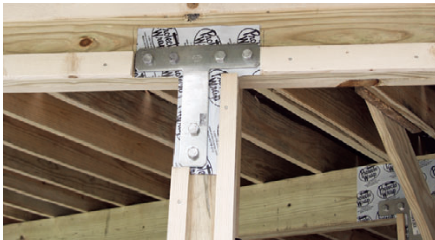
Figure 5. In cases where Y-bracing will obstruct views from doors or windows under the deck, the author substitutes rated metal T-straps at column-to-beam connections.
