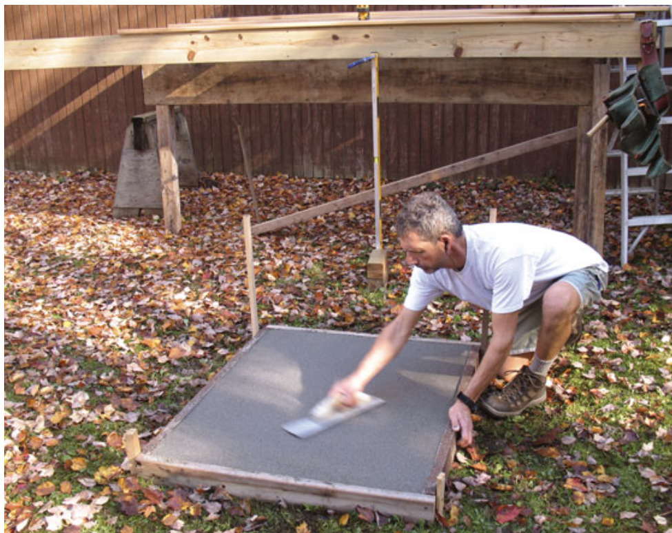
Figure 1. After making preliminary calculations to find the location of the base of the stairs, the author pours concrete for the landing.
