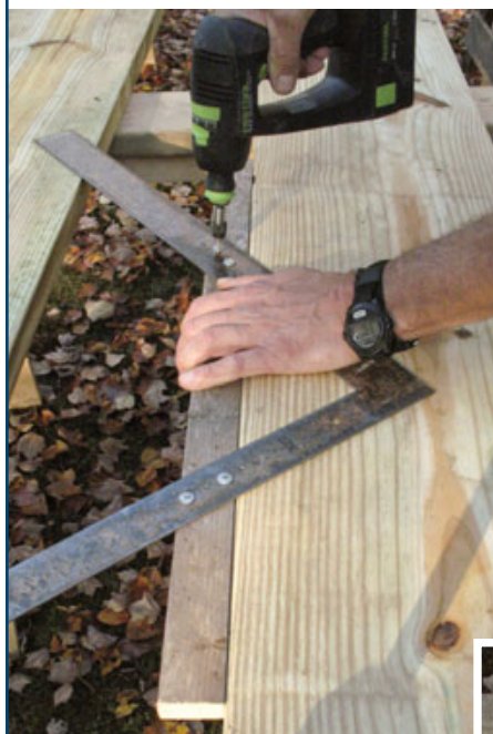
Figure 4. Rather than use stair nuts for marking out stringers, the author prefers to screw a straight 1x2 to a framing square. The 1x2 bridges any wane or other edge defects and provides a straight line that makes it easy to pinpoint riser and tread points when stepping off the stairs.
