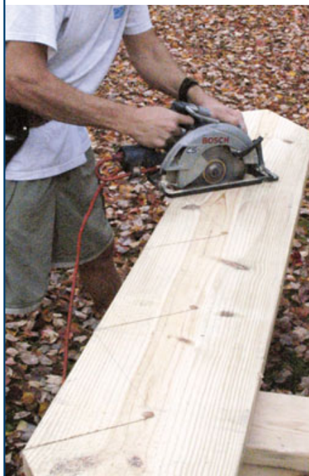
Figure 8. Making all tread cuts in succession, then cutting the risers on a second pass along the stringer, helps the author repeat a consistent entry angle for the meticulous cuts.
