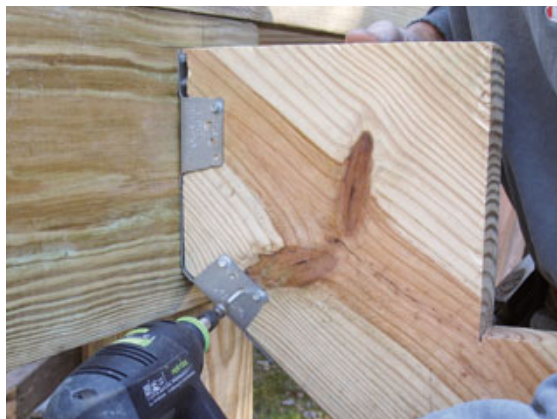
Figure 14. Use structural screws instead of nails to mount the stringer hardware. Screws are less likely to withdraw from the rim joist or header over time.
