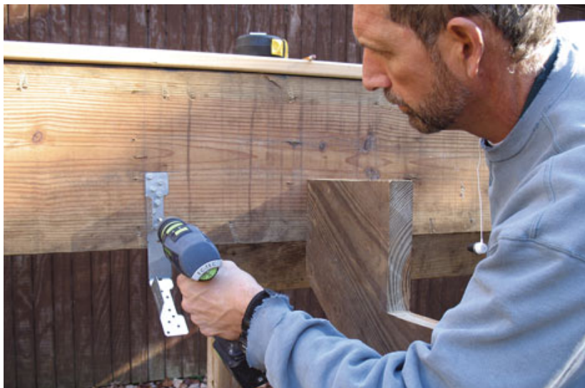
Figure 12. Only rim joists made with 2x12s (or bigger) provide enough attachment surface for use with stringer mounting brackets.
