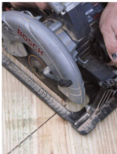
Figure 9. Stop saw cuts \frac{1}{8} inch to \frac{1}{4} inch short of the opposite lines to avoid overcutting the corners.
