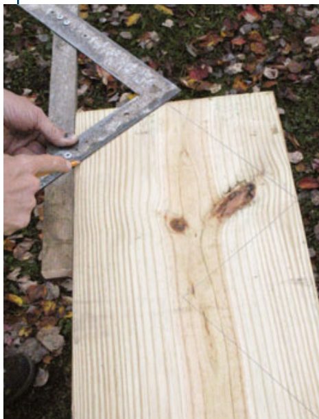
Figure 6. Mark the head cut plumb down from the back of the top tread cut.
