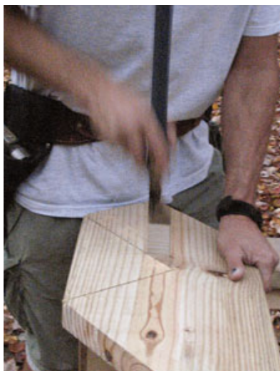
Figure 10. Finish the inside corner cuts with a handsaw, taking care not to overcut the corner.
