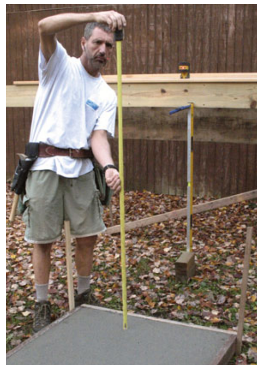
Figure 2. Use a laser level and a tape to accurately measure the total rise between the landing and the top of the finish decking.
