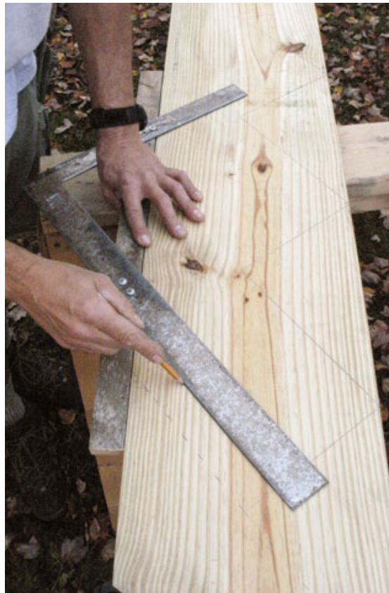
Figure 5. Mark the bottom cut on the stringer so the bottom riser is shorter than the other risers by the thickness of the tread stock. Here, the dotted line indicates the full riser height as the author marks the cut line 1\frac{1}{2} inches shorter to account for the 2x12 tread stock.
