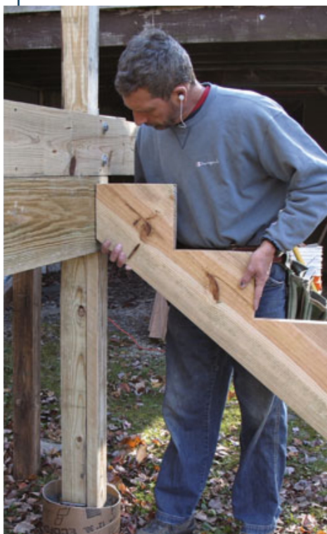
Figure 13. The author installs a structural header and support posts for the stair. The posts continue through the deck frame to support the guardrail system.
