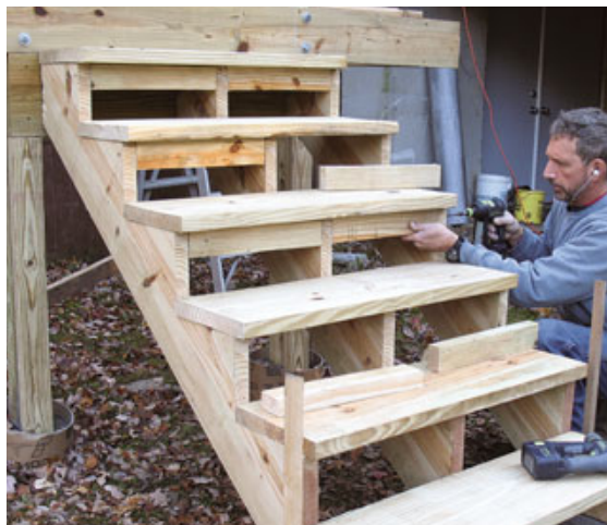
Figure 15. The open riser area must be closed down to less than 4 inches on staircases that are more than 30 inches above grade. Here the author installs ripped blocks beneath the tread above, leaving partially open risers.
