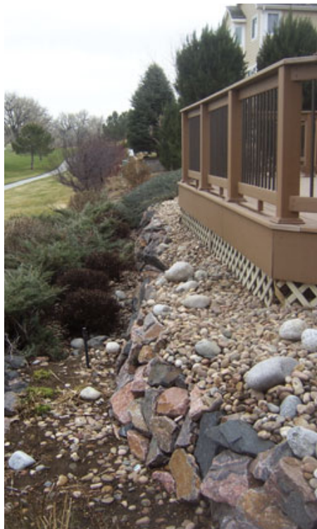
Figure 3. In previous editions of the code, rails would not have been required on this deck (left) — even though there’s an obvious fall hazard — because the grade directly next to the deck was less than 30 inches below the decking. The 2009 IRC closes this loophole, requiring that the “landing” area extend 36 inches from the edge of the deck (above).
