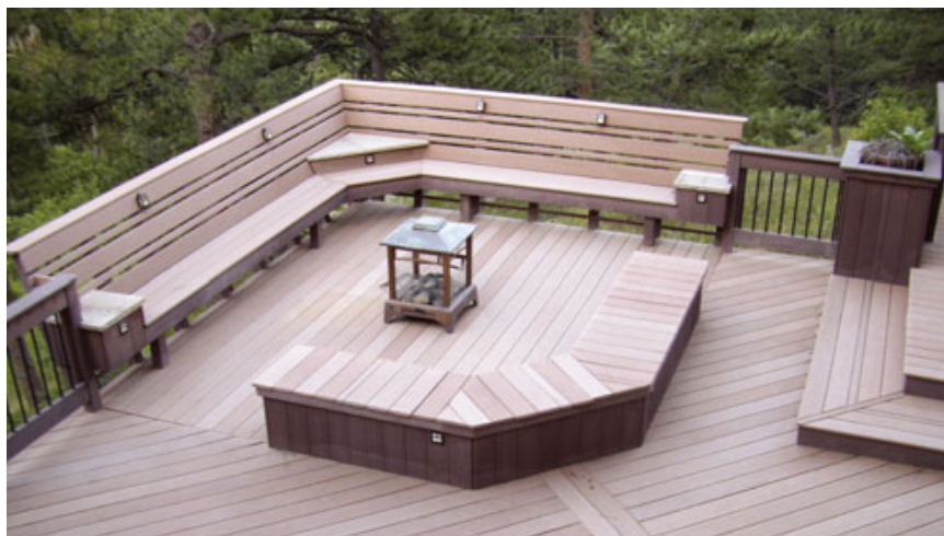
Figure 4. When this deck (above) was built under the 2003 IRC, the slanted bench-back, which is 24 inches tall, was considered a compliant guard. Under the 2009 IRC, the back of this bench would have to rise 36 inches above the seat (see illustration, top). Although the bench seat at left is higher than 30 inches above grade, the deck's walking surface is not, so no guard is required.
