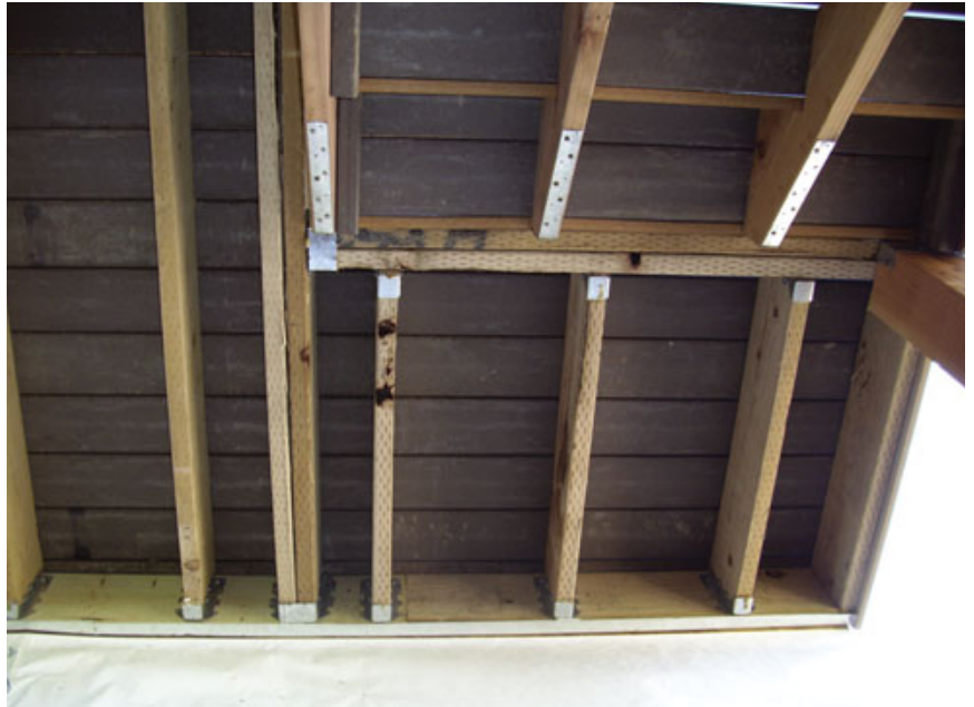
Figure 2. Because a doubled joist that supports other joists transfers a concentrated load to the ledger, it will require support beyond the code’s bolting schedule. Some inspectors will make an exception for a small stair landing, while others will prohibit all beams from loading at the ledger.
