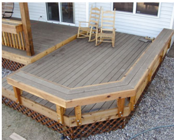
Figure 4. When this deck (above) was built under the 2003 IRC, the slanted bench-back, which is 24 inches tall, was considered a compliant guard. Under the 2009 IRC, the back of this bench would have to rise 36 inches above the seat (see illustration, top). Although the bench seat at left is higher than 30 inches above grade, the deck's walking surface is not, so no guard is required.
