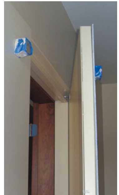
Figure 5. A closing coordinator mounted below the stop on the head jamb manages the two doors' closing sequence. The lever for the active, astragal-equipped door is mounted close to the side jamb (A, above); it holds the active door open until the passive door closes and activates a trigger mechanism located toward the center of the head jamb (B). This releases the lever holding the active door open, allowing it to close (right).
