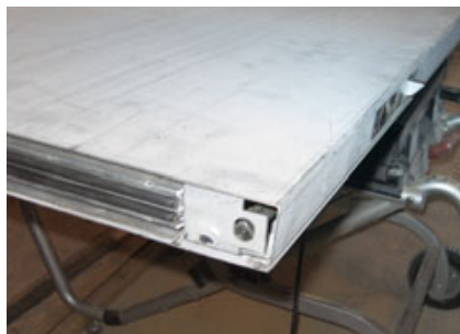
Figure 6. Adjustable flush bolts at the top and bottom of the passive door are activated by a lever mechanism in the edge of the door (left). The bolts engage when the active door closes and depresses the lever mechanism (right), then retract when the active door is opened again.
