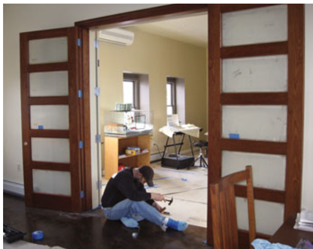
Figure 7. New wood strip flooring running diagonally through the passageway helps tie the two condo units together. The automatic fire doors maintain the integrity of the fire wall, but for daily use the owners rely on a pair of standard French doors hung on the other side of the opening.
