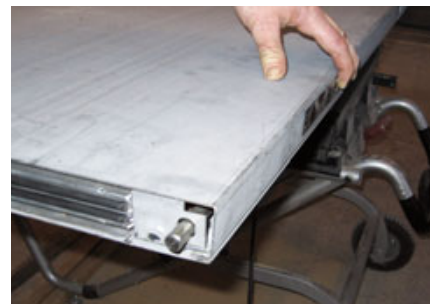
Figure 6. Adjustable flush bolts at the top and bottom of the passive door are activated by a lever mechanism in the edge of the door (left). The bolts engage when the active door closes and depresses the lever mechanism (right), then retract when the active door is opened again.
