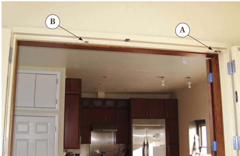
Figure 5. A closing coordinator mounted below the stop on the head jamb manages the two doors' closing sequence. The lever for the active, astragal-equipped door is mounted close to the side jamb (A, above); it holds the active door open until the passive door closes and activates a trigger mechanism located toward the center of the head jamb (B). This releases the lever holding the active door open, allowing it to close (right).
