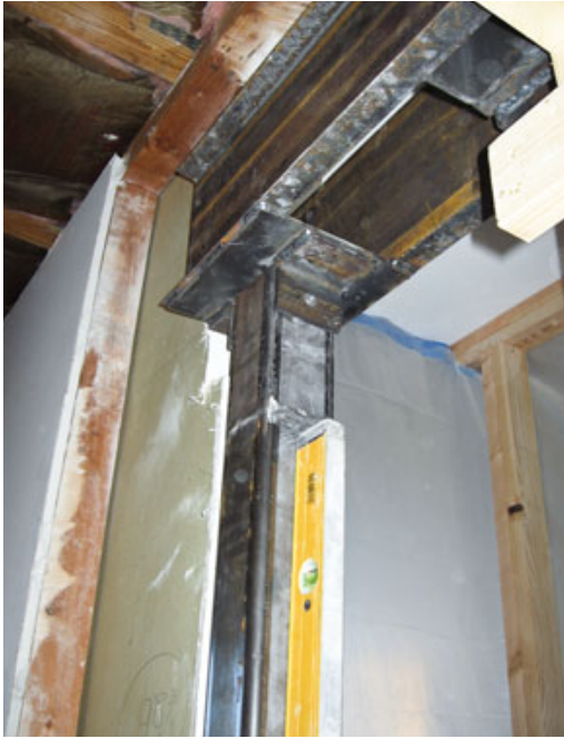
Figure 2. Two 4x4 steel columns bolted to brackets welded to the girder above provide support (left). The columns bear on the floor trusses, which are reinforced with squash blocks (right).
