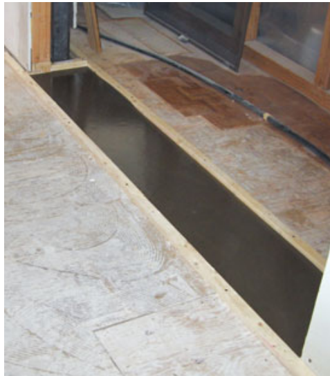
Figure 3. Fire doors can be ordered with automatic neoprene door bottoms, which seal against the floor when a plunger on the door's edge comes in contact with the jamb (above). To function properly, the door bottoms need a flat threshold, so the author's crew tacked strips of wood to the sub-floor and filled the area with self-leveling underlayment (left).
