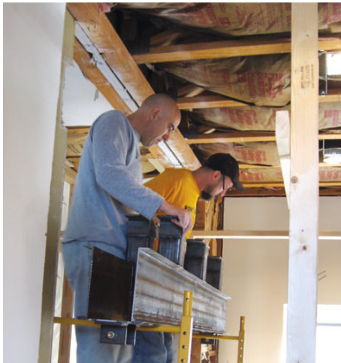
Figure 1. A custom-fabricated steel girder was required for the new opening in the double 2x4 fire wall separating the two condos (left). Pairs of steel cripples welded between steel channels support the fire wall's two top plates and the roof trusses overhead (above).
