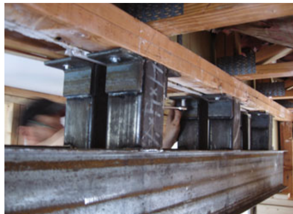
Figure 1. A custom-fabricated steel girder was required for the new opening in the double 2x4 fire wall separating the two condos (left). Pairs of steel cripples welded between steel channels support the fire wall's two top plates and the roof trusses overhead (above).
