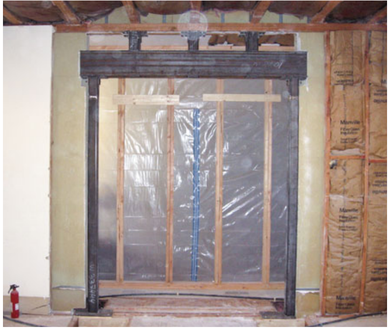
Figure 2. Two 4x4 steel columns bolted to brackets welded to the girder above provide support (left). The columns bear on the floor trusses, which are reinforced with squash blocks (right).
