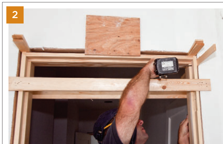
With shims at the header pinning the side jambs to the floor, the author screws the top of the hinge jamb to the framing.
