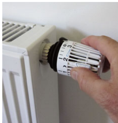
Figure 1. A thermostatic radiator valve provides room-by-room zoning for panel radiators arranged in a home-run layout. A wax-filled sensor in the valve contracts and expands in response to temperature fluctuations in the room, modulating the flow of warm water through the radiator and maintaining the desired room temperature.
