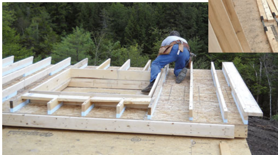
Figure 2. After framing and sheathing the 2x6 walls, the carpenters screwed 2x4s to the exterior through 2-inch foam strips and added door and window bucks (left). Lifting jacks were needed to raise the heavy walls into position (above).
