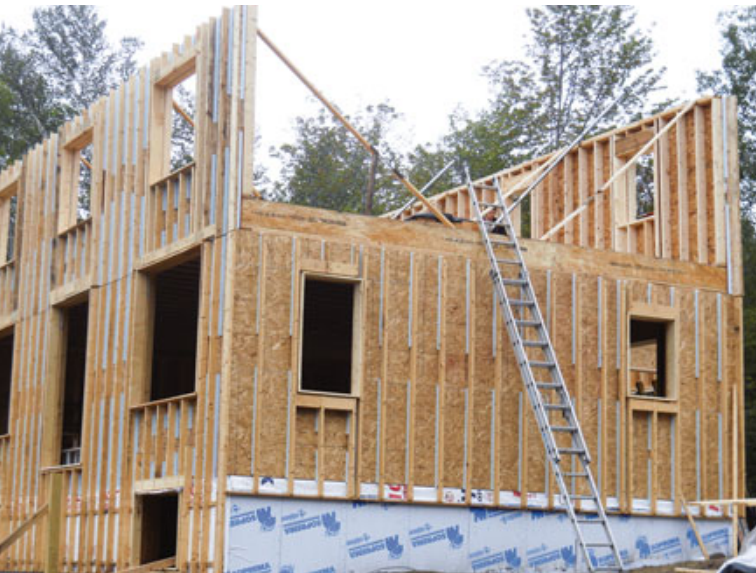
Figure 3. The exterior walls were framed so that, when lifted into place, the OSB sheathing and the outer 2x4 studs cover the rim joists (left), providing continuous bays for spray foam from the foundation to the truss top chords (below).
