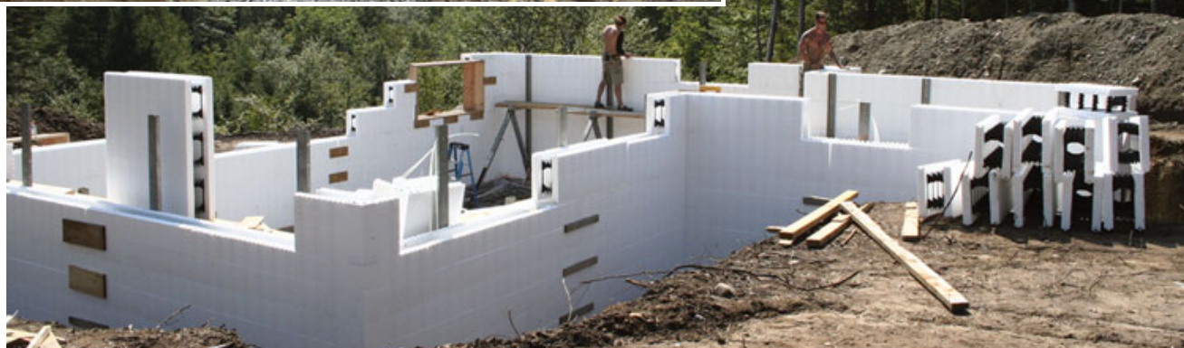
Figure 1. Fabric footing forms remain in place after the concrete is poured, creating a capillary break between the ground and the footing (top). R-26 ICF forms were used to build the foundation walls (above), which were wrapped with an additional 2-inch layer of EPS, then waterproofed with a foundation-grade peel-and-stick membrane (far left). The basement slab is insulated with two layers of 2-inch EPS foam, with a vapor barrier sandwiched in between (left).
