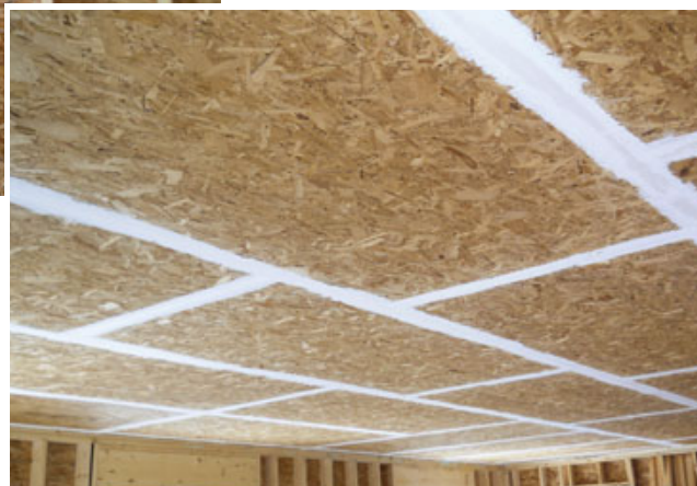
Figure 6. The truss heels and other framing joints were first air-sealed with closed-cell foam in preparation for blown-in cellulose (left). Note the site-built baffles behind the foam — pieces of plywood over strips of wood along the top chords — which allowed for 30 inches of insulation without blocking the soffit vents. To support all that cellulose, the author installed OSB rather than drywall on the bottom chords of the trusses (below). Sealed with tape and mud, the OSB provides an airtight seal between conditioned space and the attic and solid backing for the tongue-and-groove wood ceiling that followed.
