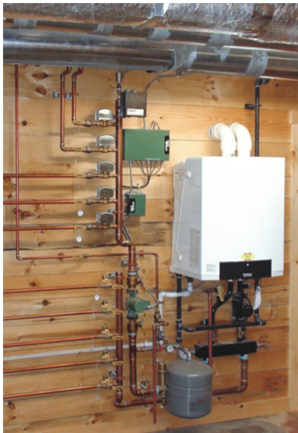
Figure 7. The home's heat is supplied by a Buderus wall-mounted propane boiler (above). The condensing unit has variable output between 22,500 and 75,000 Btu, depending on how many of the five zones are calling for heat. The 80-gallon Superstor Solar storage tank (above right) receives hot water from two roof-mounted solar thermal collectors (right); backup is provided by an electric heating element. To the left of the storage tank is a Venmar EKO 1.5 heat-recovery ventilator.
