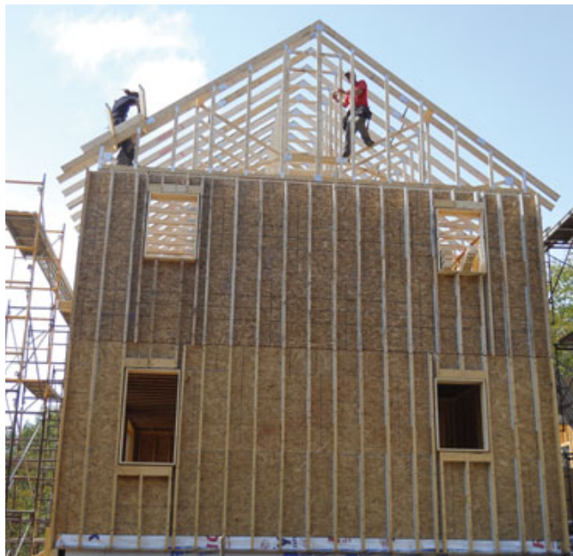
Figure 3. The exterior walls were framed so that, when lifted into place, the OSB sheathing and the outer 2x4 studs cover the rim joists (left), providing continuous bays for spray foam from the foundation to the truss top chords (below).
