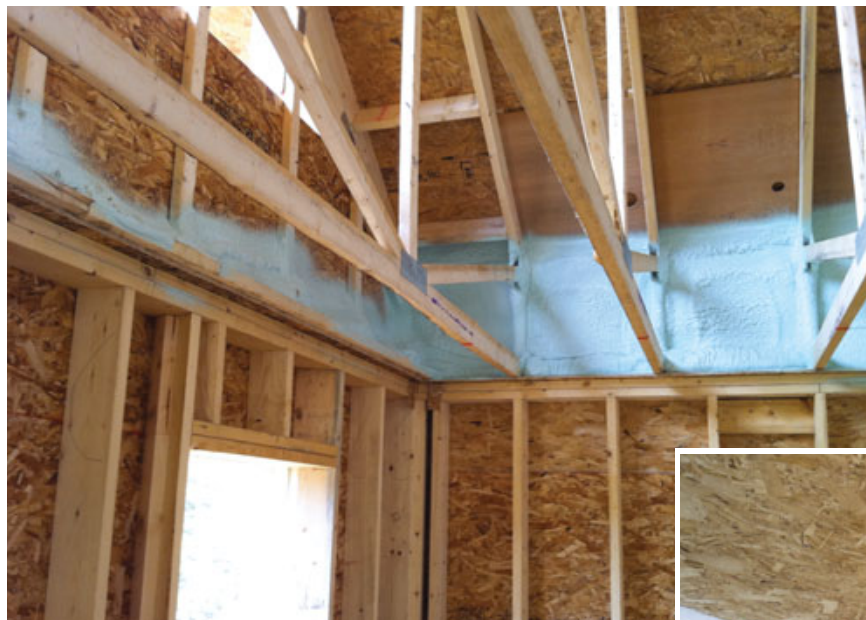
Figure 6. The truss heels and other framing joints were first air-sealed with closed-cell foam in preparation for blown-in cellulose (left). Note the site-built baffles behind the foam — pieces of plywood over strips of wood along the top chords — which allowed for 30 inches of insulation without blocking the soffit vents. To support all that cellulose, the author installed OSB rather than drywall on the bottom chords of the trusses (below). Sealed with tape and mud, the OSB provides an airtight seal between conditioned space and the attic and solid backing for the tongue-and-groove wood ceiling that followed.
