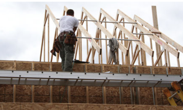
Figure 4. The roof was framed with raised-heel trusses, which allow for 24 inches of blown cellulose under the top chords at the plates (above). The trusses also have raised bottom chords down the center, creating a comfortable passageway and work platform for mechanical contractors. Dropped gable trusses support the 2½-foot-deep gable overhangs, shown here being blocked (right).
