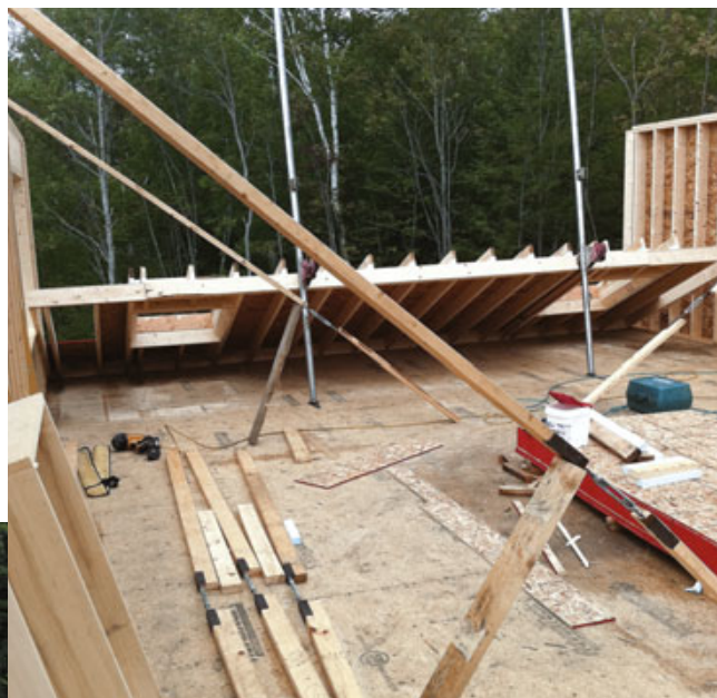
Figure 2. After framing and sheathing the 2x6 walls, the carpenters screwed 2x4s to the exterior through 2-inch foam strips and added door and window bucks (left). Lifting jacks were needed to raise the heavy walls into position (above).
