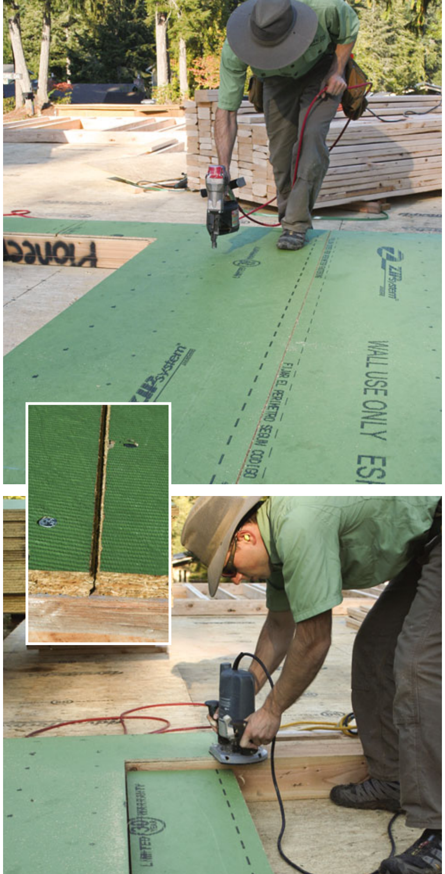
Figure 1. Zip wall panels are premarked for 16-inch and 24-inch on-center stud layouts and have a self-spacing profile along their long edges (top and inset). The author uses a router to cut out door and window openings (above); he's found that router bits tend to wear faster when cutting Zip panels than they do when cutting standard OSB sheathing, probably because of the denser material and resin-impregnated overlay.
