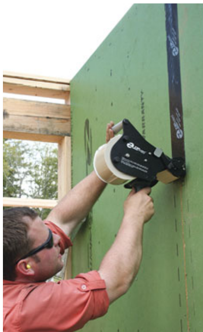
Figure 2. The author's crew uses the panel manufacturer's guns to tape seams (left). The tape gun has a built-in roller, but the crew also uses a J-roller to make sure the tape is firmly applied (top and above).
