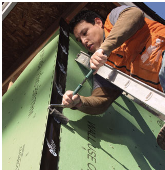
Figure 3. Corners are typically taped by hand (far left and left), though the tape gun is sometimes used for outside corners (below left). A corner tool included in the gun kit is useful for applying pressure to inside corners and valleys (below).
