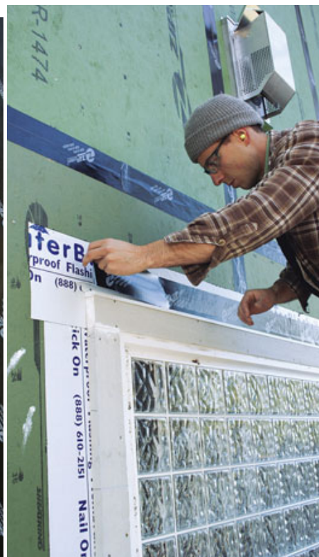
Figure 5. Either regular peel-and-stick flashing tape (left) or 6-inch-wide Zip tape can be used to flash doors and windows to the wall panels. Above, a worker seals a metal cap flashing with Zip tape.
