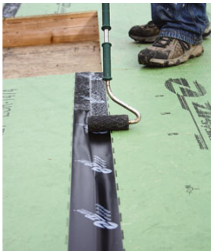
Figure 2. The author's crew uses the panel manufacturer's guns to tape seams (left). The tape gun has a built-in roller, but the crew also uses a J-roller to make sure the tape is firmly applied (top and above).
