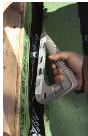
Figure 3. Corners are typically taped by hand (far left and left), though the tape gun is sometimes used for outside corners (below left). A corner tool included in the gun kit is useful for applying pressure to inside corners and valleys (below).
