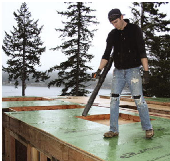
Figure 4. Zip tape can't be installed on wet surfaces, so a backpack leaf blower is used to dry off the seams in damp conditions.
