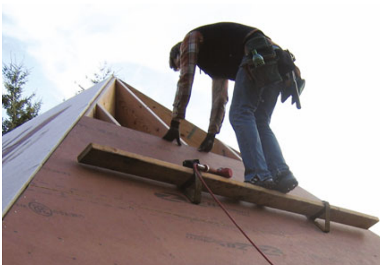
Figure 6. Zip roof panels provide good traction (left), thanks to grit added to the overlay during production. The author's crew sets up toeboards for roof pitches steeper than 8/12 (above).
