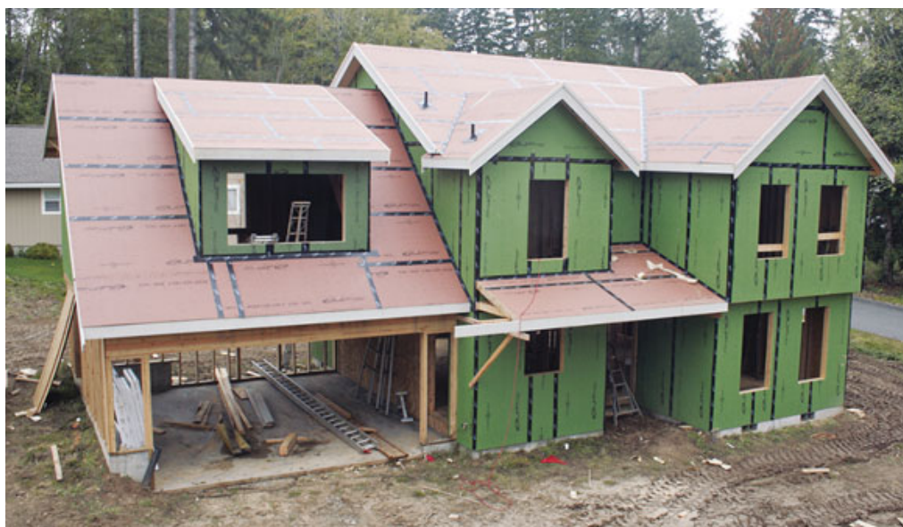
Figure 8. After the step flashing and roofing have been installed, the author tapes flashing to the sidewalls with 6-inch tape (above photos). When all the panel joints have been taped, the shell is weathertight and ready for roofing and siding (left).
