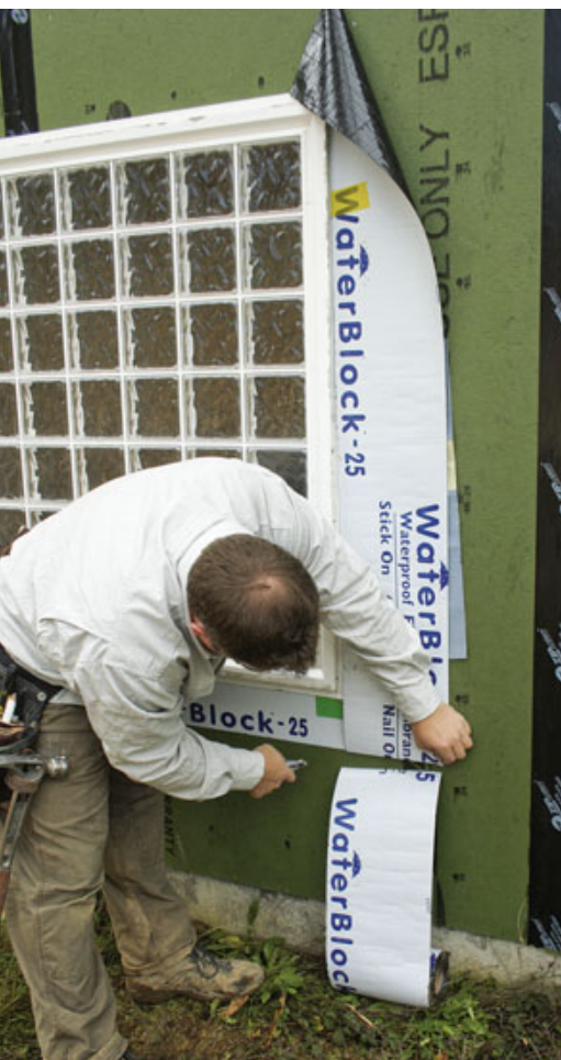
Figure 5. Either regular peel-and-stick flashing tape (left) or 6-inch-wide Zip tape can be used to flash doors and windows to the wall panels. Above, a worker seals a metal cap flashing with Zip tape.
