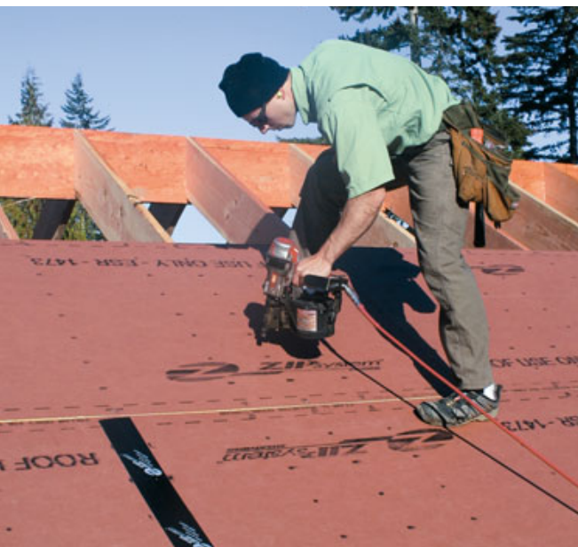
Figure 6. Zip roof panels provide good traction (left), thanks to grit added to the overlay during production. The author's crew sets up toeboards for roof pitches steeper than 8/12 (above).
