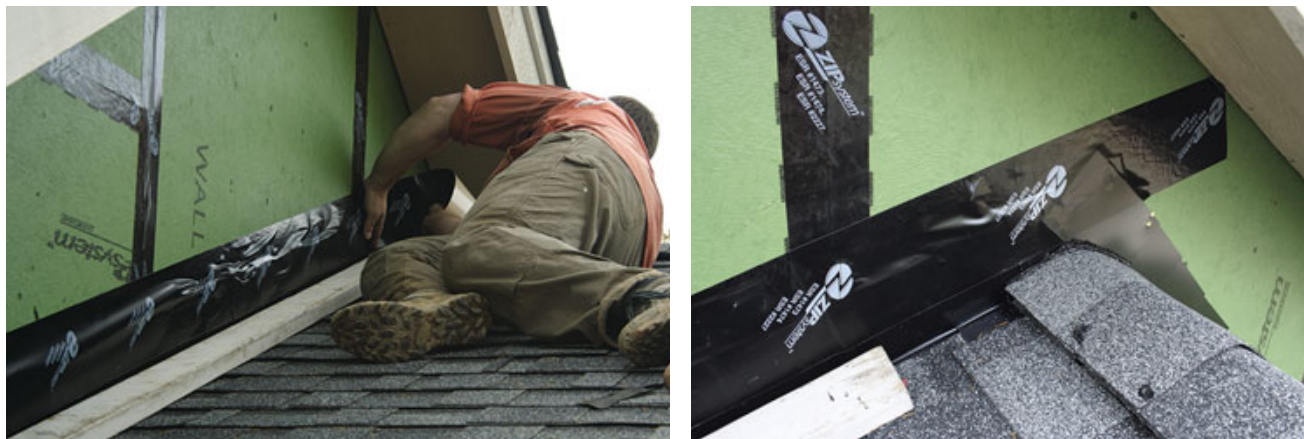
Figure 8. After the step flashing and roofing have been installed, the author tapes flashing to the sidewalls with 6-inch tape (above photos). When all the panel joints have been taped, the shell is weathertight and ready for roofing and siding (left).
