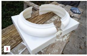
ing the splitting process will distort the column halves. In this case, we used a Turncraft column (800/423-3311, turncraft.com); the local distributor split the fiberglass column, the PVC base, and the polyurethane foam capital in its shop just before I picked up the parts and brought them to the site (2, 3).
