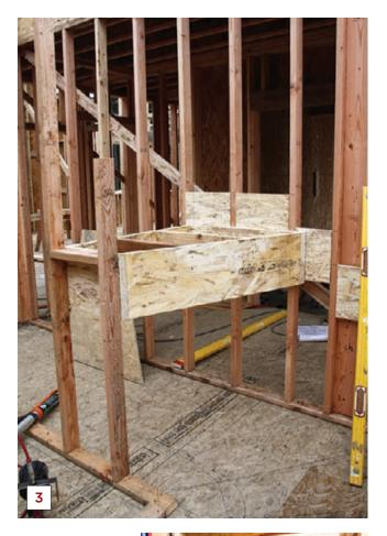
board and stiffen it with two joists (3). The other winders are open-backed; they have LSL fronts and sides, while a horizontal 2-by fastened to the riser above supports the back of the OSB treads, which I install as I go to stabilize the assembly. Vertical 2-bys add midspan support underneath (4), and everything is glued and nailed to prevent squeaks. The entire
