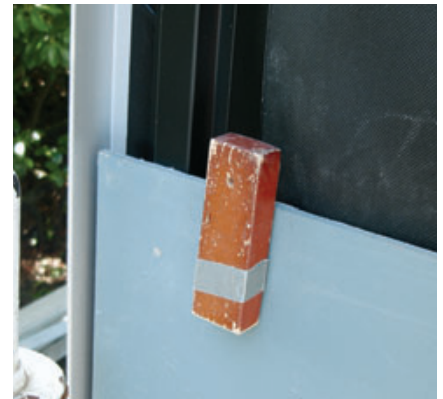
Figure 5. Horizontal panel joints are continuous around the building (left); panel layout was designed to avoid easily broken narrow ribs above or below the windows. Wooden gauge blocks were used to maintain a consistent ¼-inch spacing. Panel faces were pre-finished, and all cut edges were painted before installation (above).
