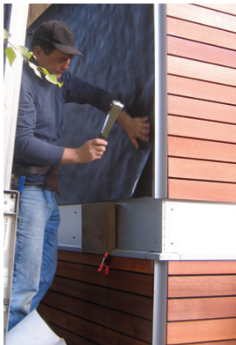
Figure 1. The open-joint method can be used with either board or panel siding. While most often used in commercial construction, it's gaining popularity in residential applications, too.
