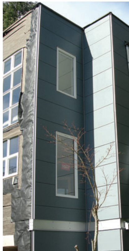
Figure 5. Horizontal panel joints are continuous around the building (left); panel layout was designed to avoid easily broken narrow ribs above or below the windows. Wooden gauge blocks were used to maintain a consistent ¼-inch spacing. Panel faces were pre-finished, and all cut edges were painted before installation (above).
