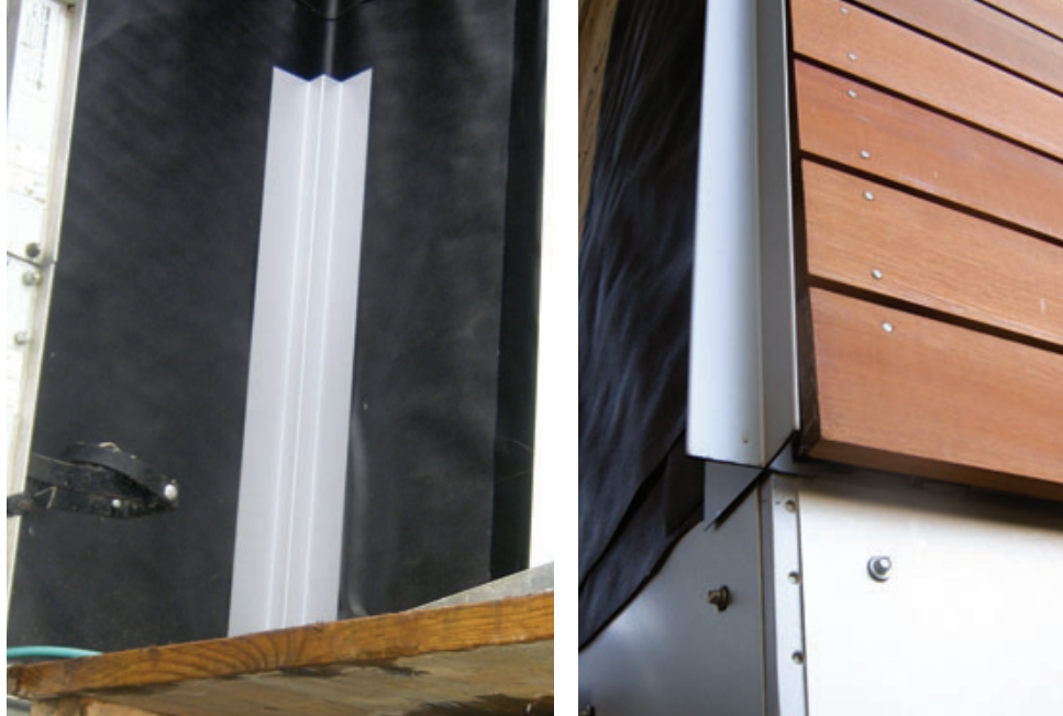
Figure 3. A custom sheet-metal shop fabricated battens and metal trim elements for the project, including inside corner trim (far left) and X-profile outside corners (left). The horizontal aluminum “belly band” was fastened to the sheathing with gasketed screws, which were driven into slightly oversized holes to allow for thermal expansion of the metal.
