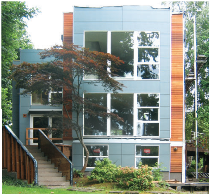
Figure 1. The open-joint method can be used with either board or panel siding. While most often used in commercial construction, it's gaining popularity in residential applications, too.
