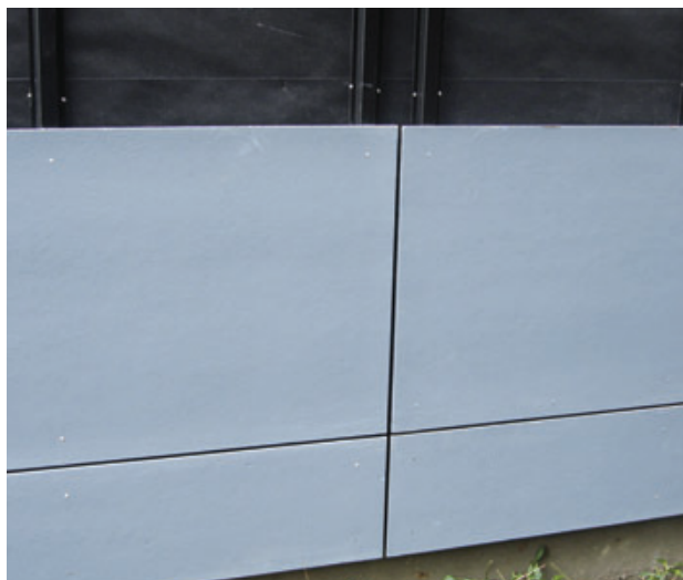
Figure 4. Fiber-cement wall panels were fastened with ring-shank stainless nails. Two battens were used at vertical joints, one on each side of the gap.
