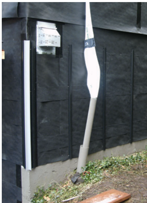
Figure 2. With narrow siding, such as these 4-inch cedar boards, two full layers of underlayment were required for UV protection (far left). Where wider panel siding was used, a full single layer was applied, followed by 6-inch strips beneath panel joints (left). The vertical “streamer” is a temporary sheet-plastic downspout.
