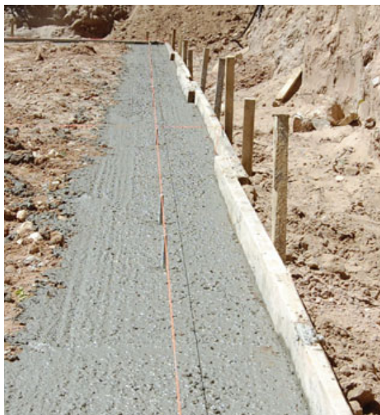
Figure 2. Although wood foundations have traditionally been supported by footings of carefully compacted gravel or crushed stone, a poured concrete strip footing (left) can also be used. The poured footing simplifies the process of snapping layout lines and provides a convenient surface for marking plates and assembling wall framing (below).
