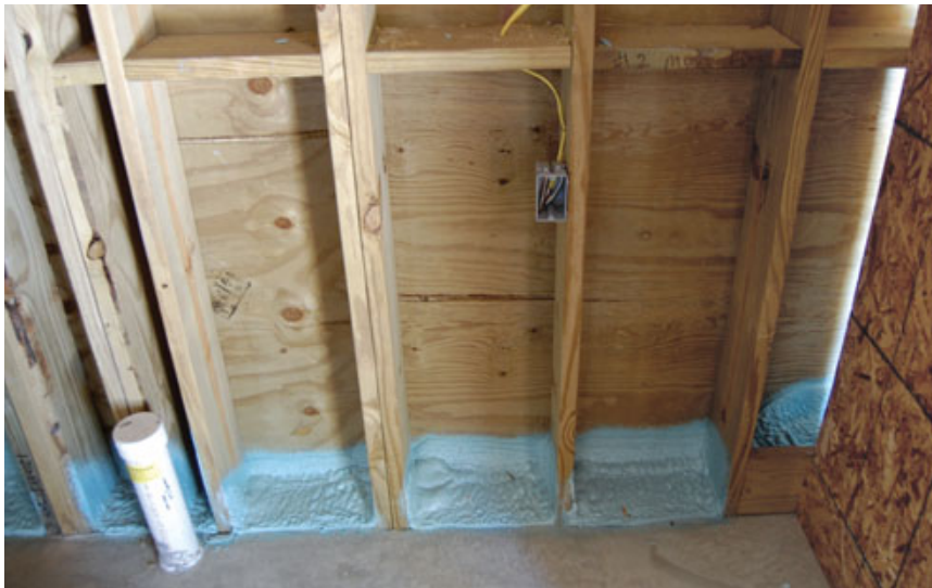
Figure 5. Targeted applications of spray foam air-seal and insulate the rim joists (left) and the bottom plates (below), where scraps of OSB were laid down to protect the slab floor from overspray. Damp-spray cellulose insulates the stud cavities (bottom).
