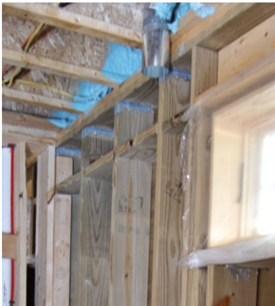
Figure 5. Targeted applications of spray foam air-seal and insulate the rim joists (left) and the bottom plates (below), where scraps of OSB were laid down to protect the slab floor from overspray. Damp-spray cellulose insulates the stud cavities (bottom).
