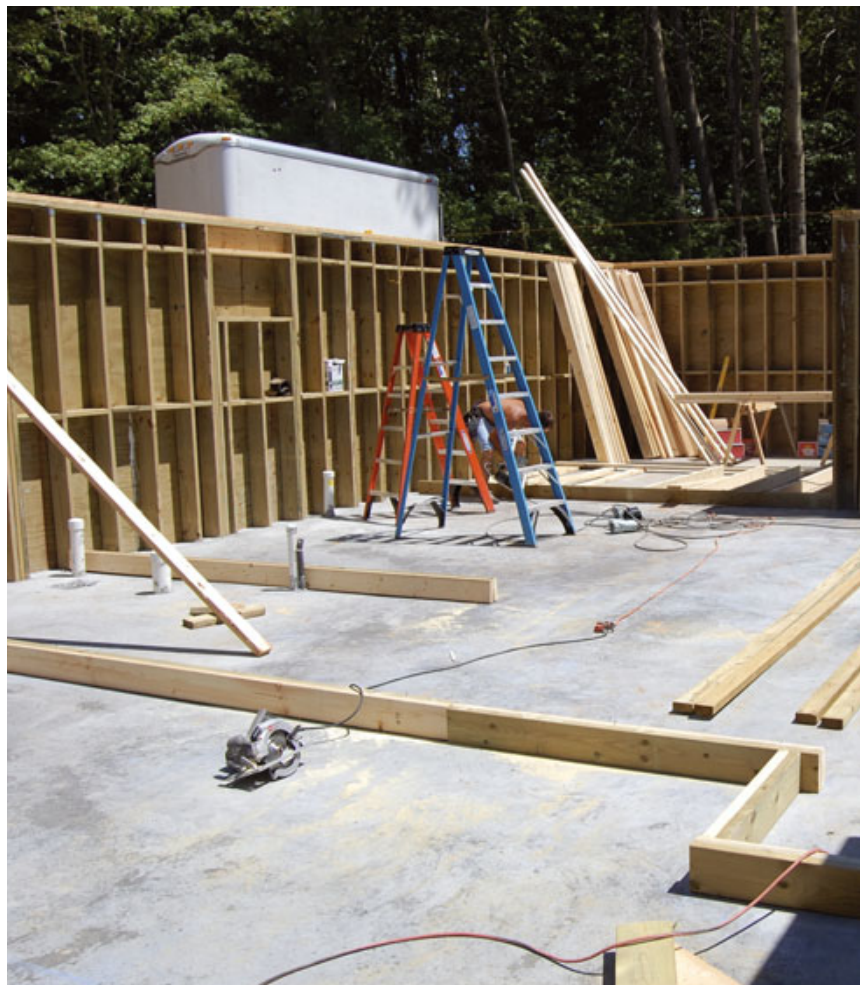
Figure 4. Once the basement slab has been poured and finished (above), shear walls and partitions can be erected. Two partially sheathed shear walls are visible here (right), each of which extends from the long wall at right to an inside corner at left. A doubled I-joist at the top plates (indicated in photo by dotted red lines) will provide a solid connection between the shear walls and the floor diaphragm overhead.
