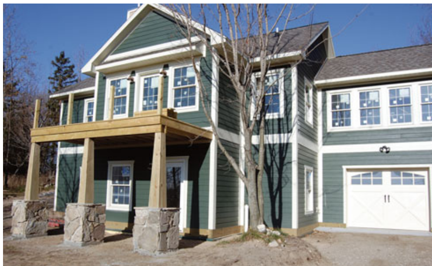
Figure 6. Before the excavation is backfilled, the below-grade portion of the exterior is wrapped with 6-mil poly (top left), the top of which will be secured to the wall with a pressure-treated grade board. On the sided building, the grade board is carried along the sidewall (top right) and across the walkout front (above).
