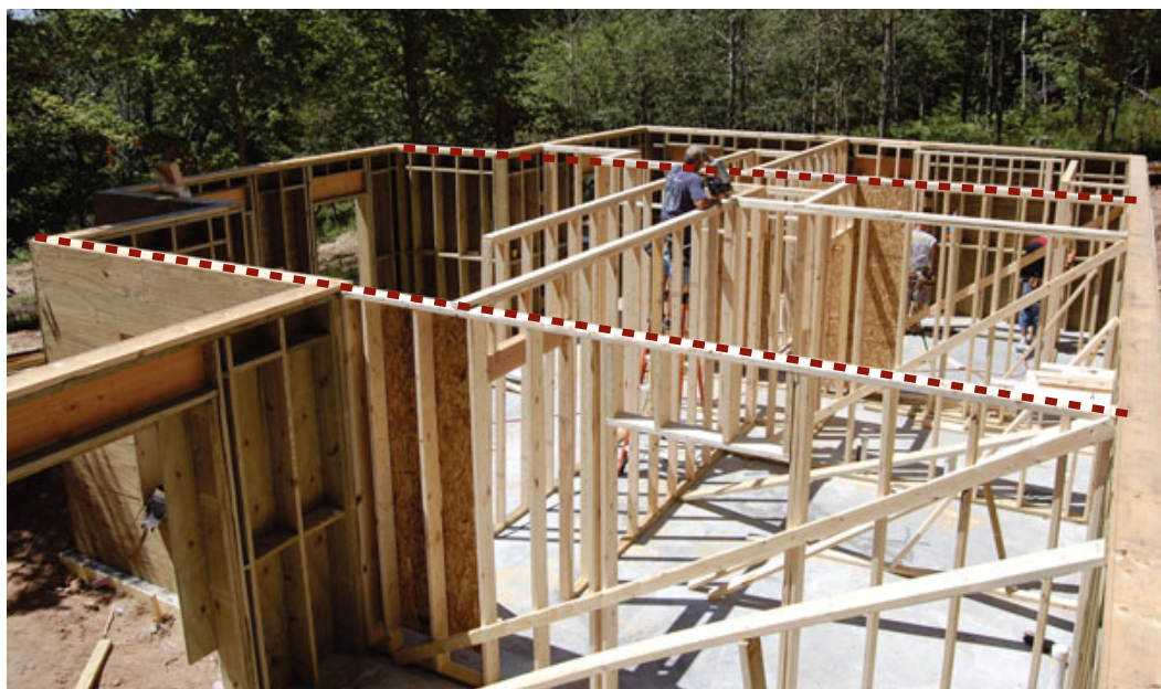
Figure 4. Once the basement slab has been poured and finished (above), shear walls and partitions can be erected. Two partially sheathed shear walls are visible here (right), each of which extends from the long wall at right to an inside corner at left. A doubled I-joist at the top plates (indicated in photo by dotted red lines) will provide a solid connection between the shear walls and the floor diaphragm overhead.
