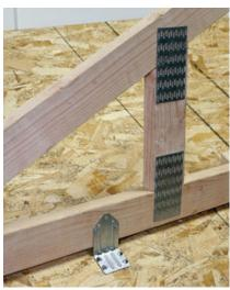
porting roof. The maker says that the truss can be set first and the connector added after the crane has been sent on its way. You can fasten the clip with nails, but if greater uplift resistance is needed Strong-Drive SD screws are recommended. The VTCR connector can accommodate pitches up to 12/12. It costs about \$2.25.
