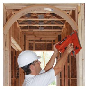
Prefab Arches. Want to avoid the hassle of fabricating curved framing on site? Consider sending the plans to *Custom-Arch* and letting someone else do the work. This company makes solid wood framing arches for interior and exterior uses — everything from single curves for arch-top windows and doors to complex domes and groin vaults. It says it can bend arches down to an 8-inch radius and span widths greater than 20 feet. A single 3/0 arched doorway costs about \$25 (not including installation).
