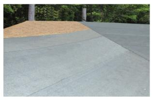
Modern Membrane. *IB-3 StormStopper* is a self-adhering (50-mil-thick) mineral surface underlayment that can be used to protect trouble spots like valleys and rake edges or the entire roof. Made with a rubberized asphalt adhesive that self-seals around fasteners and projections, the liner separates easily and splits in the middle to simplify valley installations, says the maker. It comes in 3-foot-by-67-foot rolls. The company declined to provide pricing.
