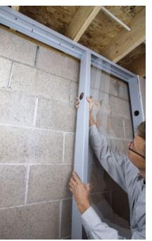
Plastic Studs. The EcoStud Track and Stud System for framing basement walls assembles like steel studs but doesn't have steel's thermal conductivity problems. The 100 percent recycled plastic material fastens with standard drywall screws (though the company recommends also using adhesive to fasten drywall). Prepunched slots in the track lock studs in place. An 8-foot stud costs about \$5.
