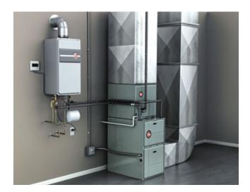
Forced Air and Hot Water. Plenty of hydronic systems use the same boiler for heat and hot water, but few provide cooling as well. Rheem's Integrated HVAC & Water Heating System uses a tankless water heater as a boiler, heats forced air with a hydronic air handler, and can be combined with various cooling coils and plenums to complete an hvac system. Pricing for the full package (hvac and hot water) ranges from \$1,850 to \$4,550.
