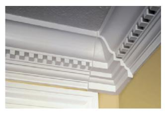
Simplified Crown. Not everyone relishes the challenge of coping and mitering crown molding. If you just want to get the job done, consider Fypon's *Miterless Crown Moulding*. The company sells a variety of lightweight one-piece urethane moldings in lengths up to 16 feet, as well as premitered inside and outside corner pieces and divider blocks that eliminate the need for scarf joints. Moldings run about \$6 per lineal foot; inside and outside corners cost about \$13 per piece.
