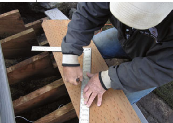
Figure 9. Mark the riser cuts using a square that's aligned with the tread cut below and the mark representing the front of the tread run above.
