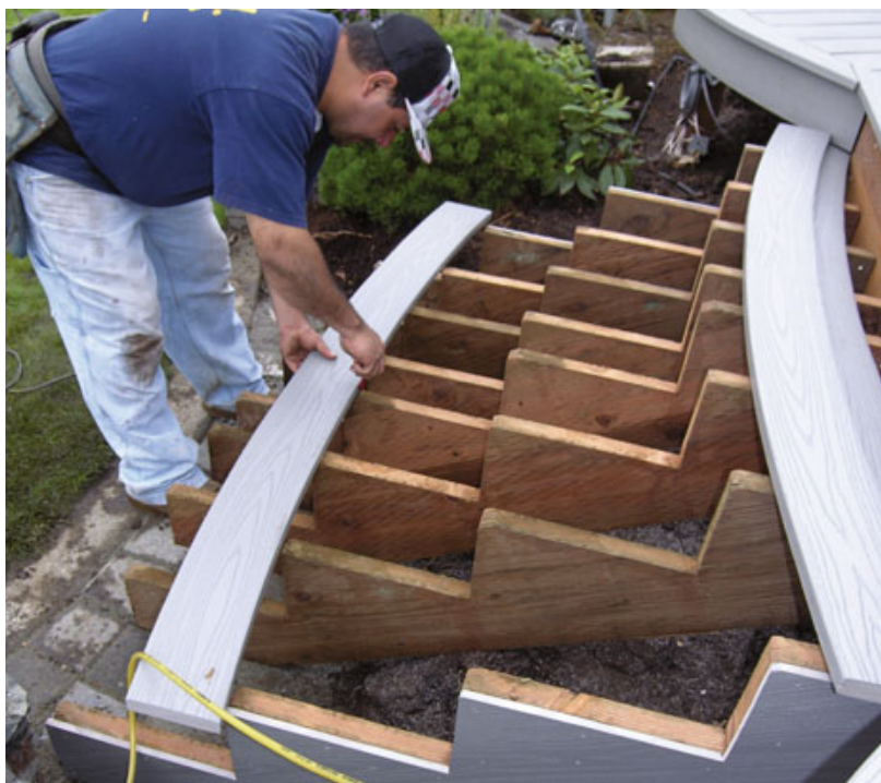
Figure 11. Complete the stair by installing the risers and the tread stock.
