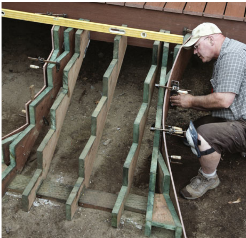
Figure 10. Thin deck fascia is shimmed out from the top and bottom of the diagonal jack to establish the flare.
