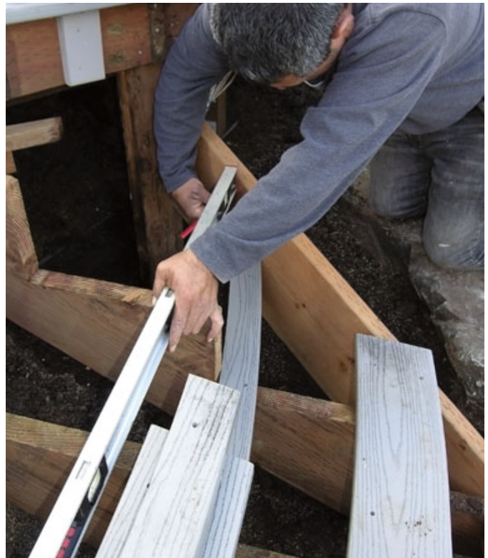
Figure 8. A level placed across the main jacks is used to establish the tread elevations on the diagonal jacks.
