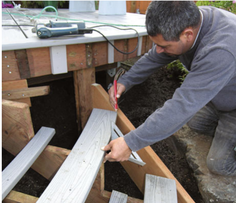
Figure 6. Verify the diagonal jack's location with a piece of bent decking or a plywood tread template.
