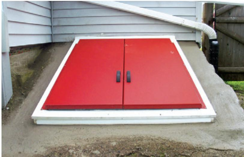
Proper flashing and a solid base of pressure-treated lumber and cellular PVC promise long life
