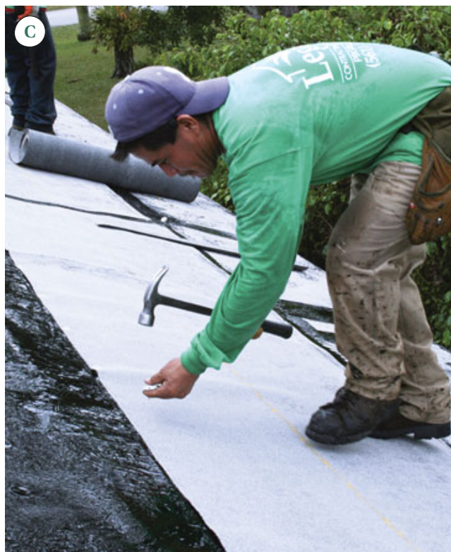
Figure 4. Before hot mopping begins, a roofer coats metal valley flashings with asphalt primer (A). The hot tar is spread one course of asphalt roofing at a time (B), and then the 90-pound membrane is quickly applied before the tar cools. A row of metal cap nails along the top edge holds the felt in place while the asphalt cools and cures (C).
