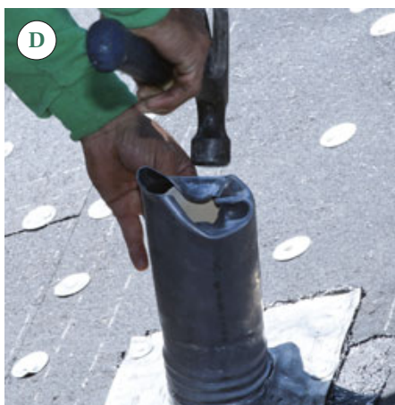
Figure 3. A reroof job usually includes new self-flashing skylights with integral curbs. A roofer applies cold asphalt cement to the new asphalt felt paper (A), sets the skylight into the tar, and secures it with ring-shank nails (B). Vent stacks are sealed with prefabricated lead flashings (C), which are set in asphalt cement, nailed off, and bent around the top of the pipe (D).
