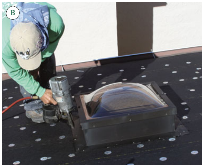
Figure 3. A reroof job usually includes new self-flashing skylights with integral curbs. A roofer applies cold asphalt cement to the new asphalt felt paper (A), sets the skylight into the tar, and secures it with ring-shank nails (B). Vent stacks are sealed with prefabricated lead flashings (C), which are set in asphalt cement, nailed off, and bent around the top of the pipe (D).
