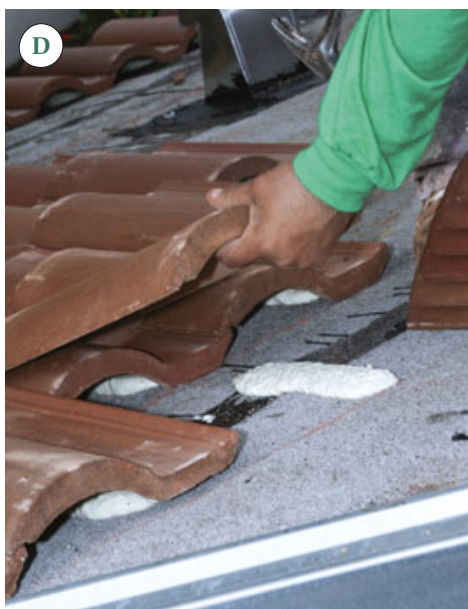
Figure 5. At roof edges, the crew attaches the cement tiles using redundant methods: a thick dab of two-part polyurethane adhesive foam (A), plus two galvanized screws per tile (B), driven through a strip of cold-applied asphalt cement. In the field, only the foam is used (C, D), to avoid screw holes in the newly applied hot-mopped underlayment.
