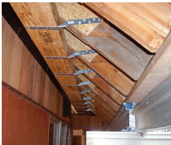
Figure 2. Six steel tie rods connect the horizontal glulam beam at the exterior wall top plate to the floor diaphragm beneath the balcony (above). The beam is attached with twist straps to AdvanTech gussets nailed to the sides of the rafters (left). Part of the beam is in the exterior soffit and part of it is inside the 20-foot box bay (below).
