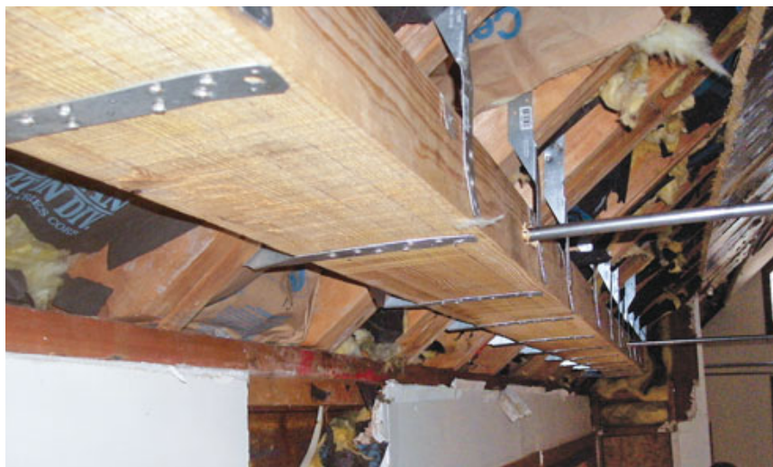
Figure 2. Six steel tie rods connect the horizontal glulam beam at the exterior wall top plate to the floor diaphragm beneath the balcony (above). The beam is attached with twist straps to AdvanTech gussets nailed to the sides of the rafters (left). Part of the beam is in the exterior soffit and part of it is inside the 20-foot box bay (below).
