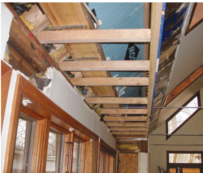
Figure 4. Hurricane clips tie the rafters to the floor joists at the front of the house; shown here is a section of the attic behind a knee wall (top). A new soffit hides the horizontal glulam beam where it runs through the cathedral bump-out (above); the tie rods were later hidden in false pine beams.
