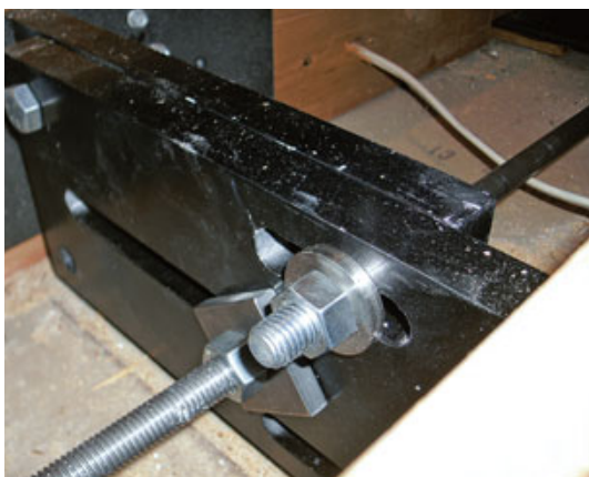
Figure 3. Heavy steel H-brackets installed between the second-story floor joists receive the interior ends of the tie rods (above and left). The two-part brackets have sliding adjustment slots to allow for variation in the width of the joist bays. Because the weight of the roof was being carried by scaffolding, nylon ratchet straps (below) hooked to the steel brackets were sufficient for pulling in the leaning wall.
