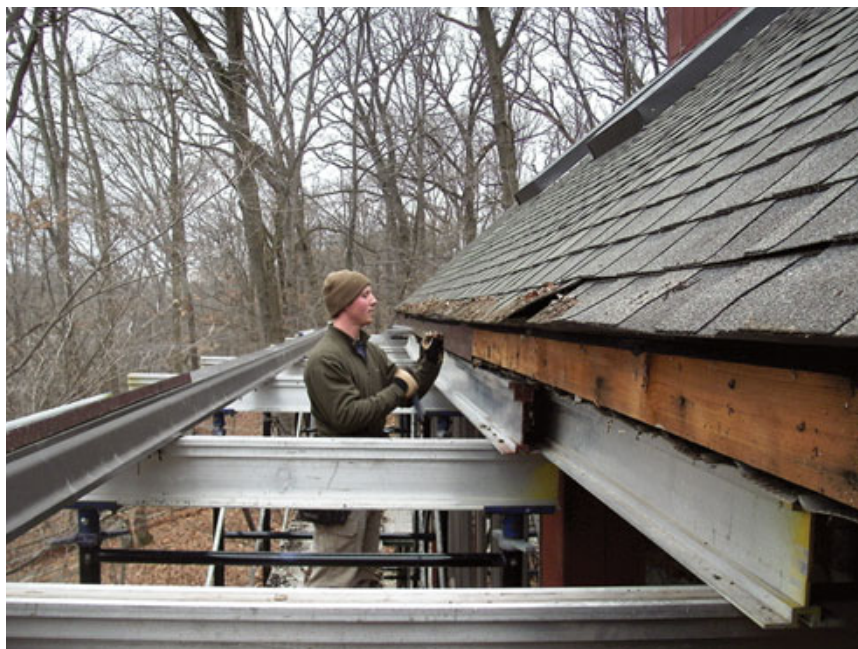
Figure 1. Heavy-duty pipe staging (top) equipped with steel cradles (above) supported a grid of aluminum I-beams used to lift the rafters off the wall. Shoring jacks at the base and adjustment screws at each cradle allowed the roof to be raised carefully and remain level.
