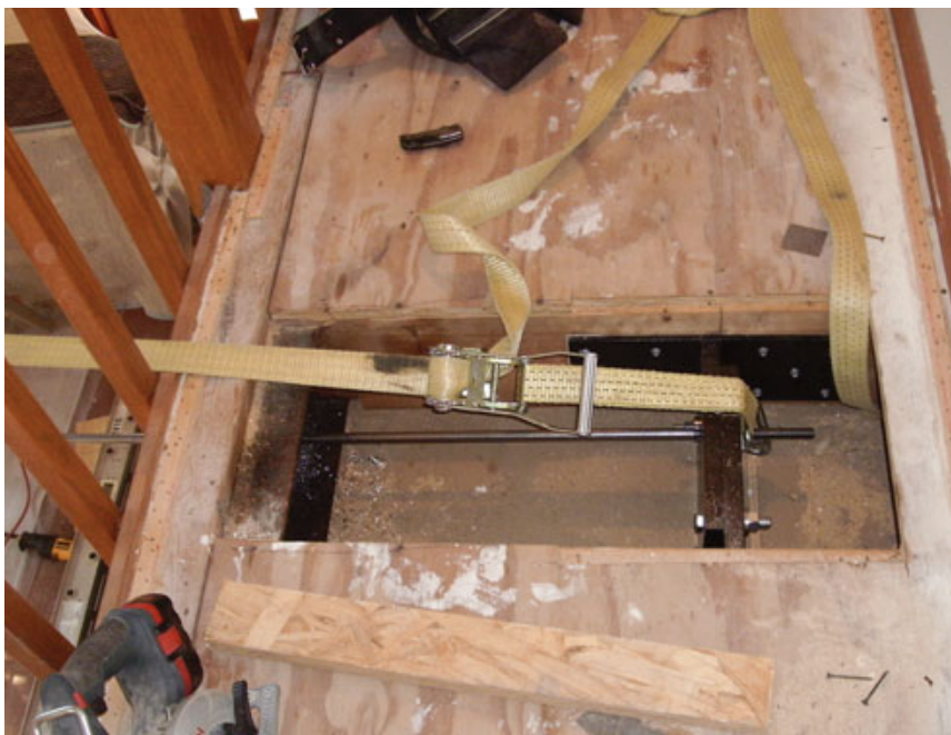
Figure 3. Heavy steel H-brackets installed between the second-story floor joists receive the interior ends of the tie rods (above and left). The two-part brackets have sliding adjustment slots to allow for variation in the width of the joist bays. Because the weight of the roof was being carried by scaffolding, nylon ratchet straps (below) hooked to the steel brackets were sufficient for pulling in the leaning wall.
