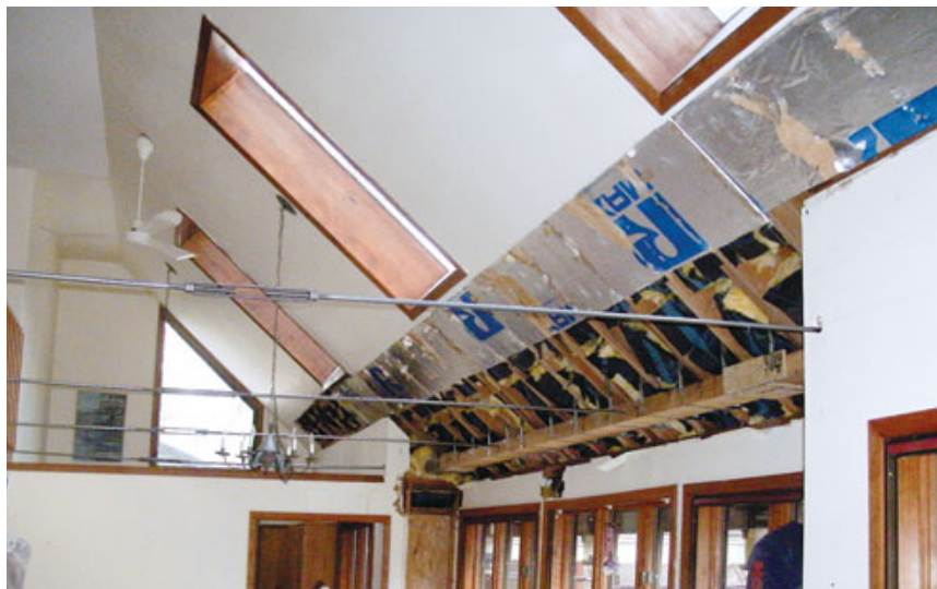
Figure 2. Six steel tie rods connect the horizontal glulam beam at the exterior wall top plate to the floor diaphragm beneath the balcony (above). The beam is attached with twist straps to AdvanTech gussets nailed to the sides of the rafters (left). Part of the beam is in the exterior soffit and part of it is inside the 20-foot box bay (below).
