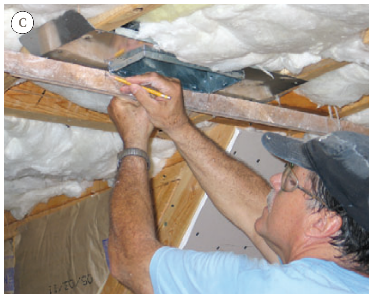
Figure 2. Rigid rulers are good for taking ceiling measurements because they don't collapse (A). On this project, the author also used a 144-inch-long story pole as a measuring stick (B) and to record the location of openings that had to be cut into the panels (C). A Gomito universal carpenter's square clamped to the panel acts as a stop for the measuring stick (D).
