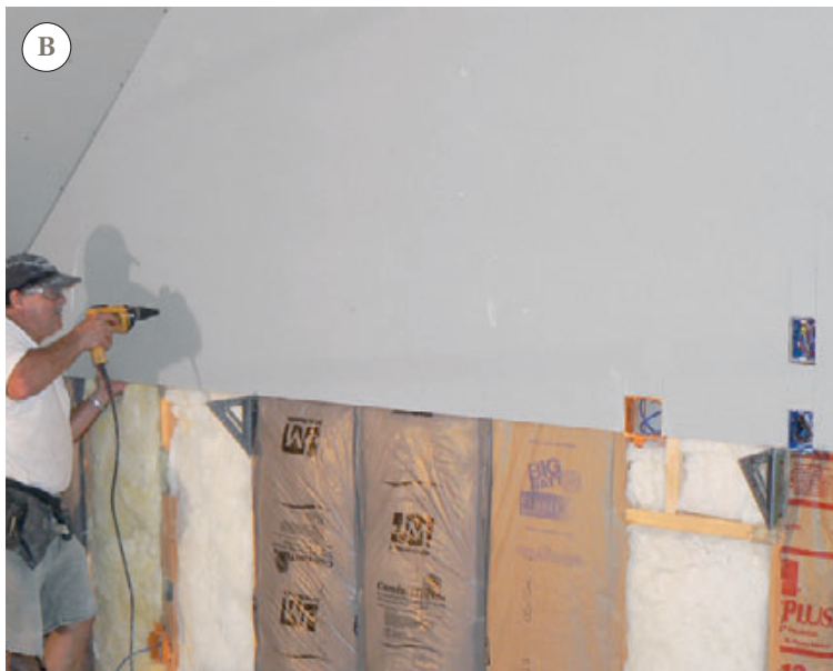
Figure 5. Swanson MAG squares — modified with holes drilled through their fences so that they can be screwed to the framing — make handy support brackets for panels (A). The author installs the upper course first, locating the brackets about 48\frac{3}{8} inches below the ceiling (B). The brackets can also be used for small ceiling sections, in places where a panel lift won't fit (C).
