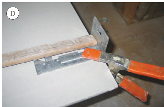
Figure 2. Rigid rulers are good for taking ceiling measurements because they don't collapse (A). On this project, the author also used a 144-inch-long story pole as a measuring stick (B) and to record the location of openings that had to be cut into the panels (C). A Gomito universal carpenter's square clamped to the panel acts as a stop for the measuring stick (D).
