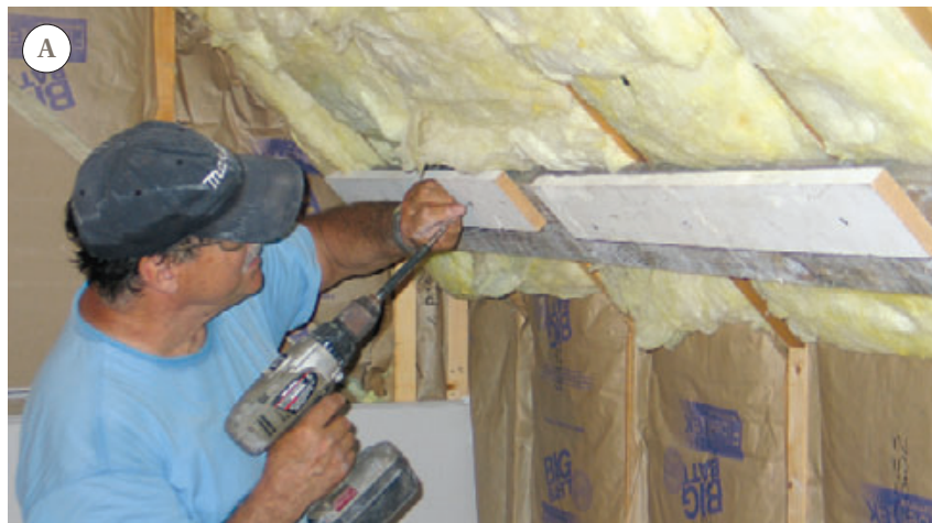
Figure 6. Before installing drywall on a sloped ceiling, the author fastens a simple cleat made from scrap lumber to the framing about 48 3 / 8 inches below the wall/ceiling junction (A). The cleat supports the lower edge of the drywall, allowing him to align the sheet with one hand while driving screws into the framing with the other (B). With tall sloped ceilings that require two full courses of drywall, the author fastens a 1-by cleat to the bottom edge of the upper sheet with a single screw, then rotates the cleat to lock the lower sheet in place (C).
