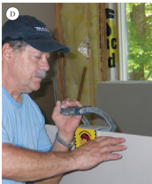
Figure 1. Whenever possible, the author works off the stack of stocked drywall (A); otherwise, he uses two 18-inch-high benches as a work platform, tilting each panel against their ends and then dragging it on top (B). From that height, lifting the cut panel is a lot easier (C) than it would be from the floor. A Gorilla Gripper — an aluminum handle that clamps to the board's top edge (D) — is helpful for moving large pieces.
