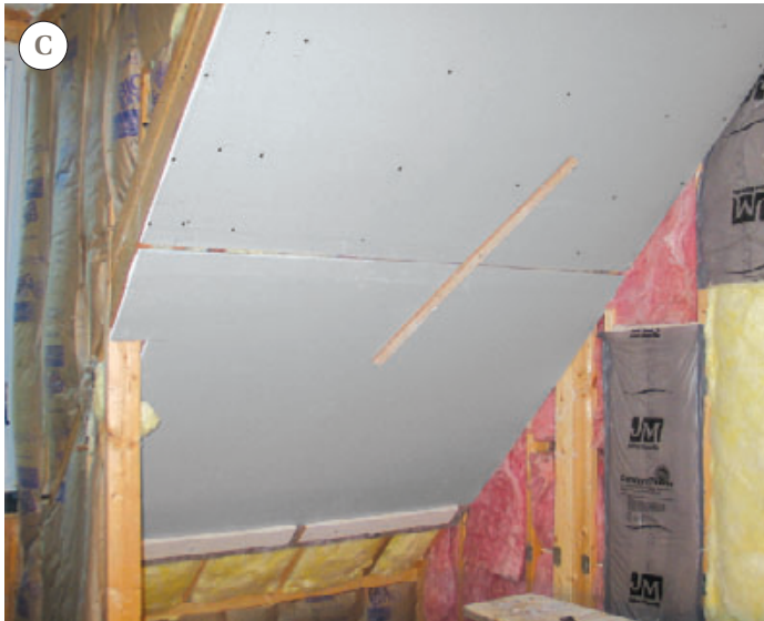
Figure 6. Before installing drywall on a sloped ceiling, the author fastens a simple cleat made from scrap lumber to the framing about 48 3 / 8 inches below the wall/ceiling junction (A). The cleat supports the lower edge of the drywall, allowing him to align the sheet with one hand while driving screws into the framing with the other (B). With tall sloped ceilings that require two full courses of drywall, the author fastens a 1-by cleat to the bottom edge of the upper sheet with a single screw, then rotates the cleat to lock the lower sheet in place (C).
