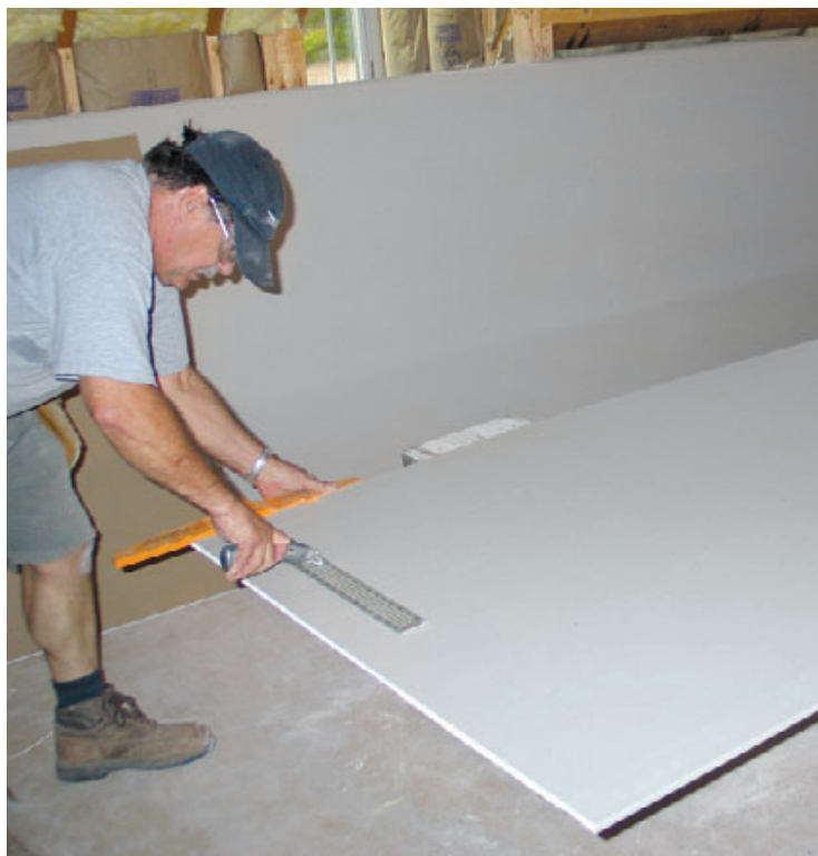
Figure 3. The author makes long parallel rips with the help of a Johnson RockRipper scoring square (left). To lay out irregular cuts, he either fastens a straightedge to the panel with spring clamps or snaps a chalk line, making a short kerf in the panel to hold one end of the line (above).
