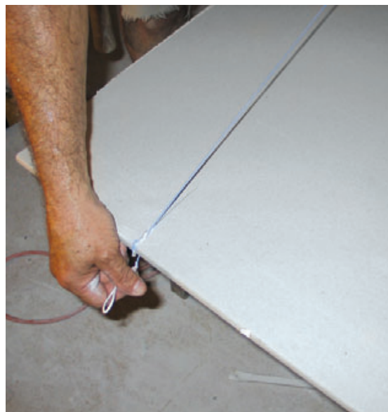
Figure 3. The author makes long parallel rips with the help of a Johnson RockRipper scoring square (left). To lay out irregular cuts, he either fastens a straightedge to the panel with spring clamps or snaps a chalk line, making a short kerf in the panel to hold one end of the line (above).
