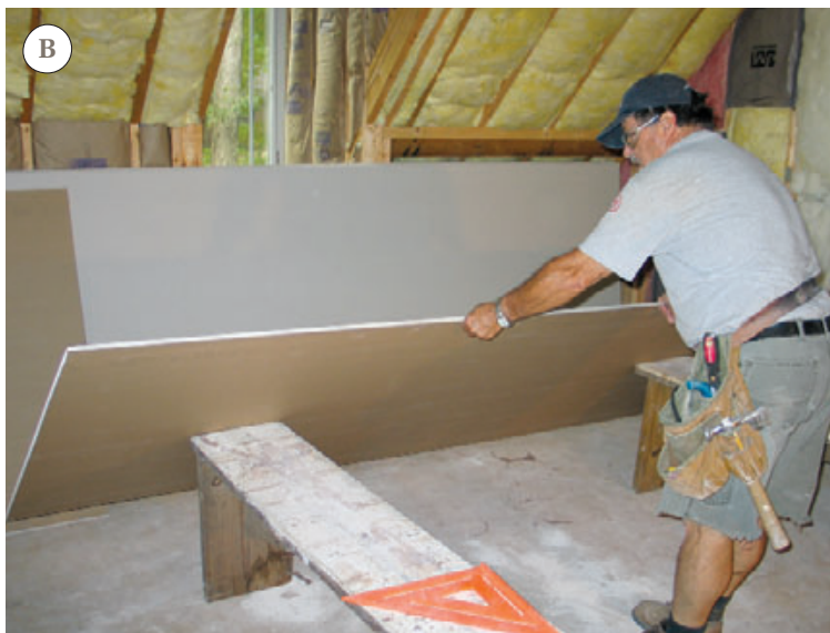
Figure 1. Whenever possible, the author works off the stack of stocked drywall (A); otherwise, he uses two 18-inch-high benches as a work platform, tilting each panel against their ends and then dragging it on top (B). From that height, lifting the cut panel is a lot easier (C) than it would be from the floor. A Gorilla Gripper — an aluminum handle that clamps to the board's top edge (D) — is helpful for moving large pieces.
