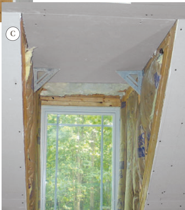
Figure 5. Swanson MAG squares — modified with holes drilled through their fences so that they can be screwed to the framing — make handy support brackets for panels (A). The author installs the upper course first, locating the brackets about 48\frac{3}{8} inches below the ceiling (B). The brackets can also be used for small ceiling sections, in places where a panel lift won't fit (C).
