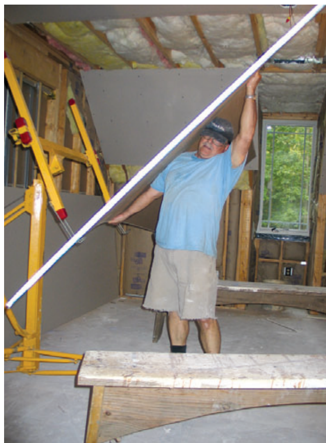
Figure 4. Instead of trying to hoist sheets straight up and into the Telpro panel lift, the author tilts them until their bottom edge clears the lift's support hooks.
