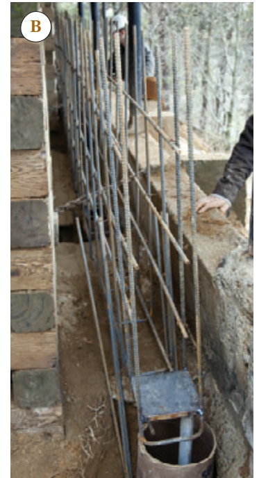
Figure 6. Heavy steel bearing plates welded to the tops of the piers support a beefy rebar cage, which has been spot-welded to the plates (A). Tube forms surround the upper ends of the piers, to encase them in concrete (B). After the last welds are made (C), the grade beam is ready to be poured (D).
