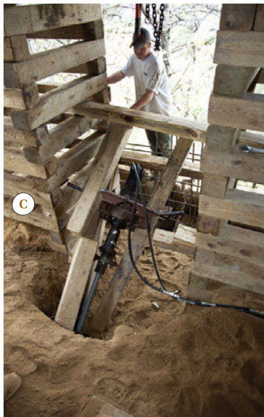
Figure 5. As the required driving force increased (A), a drag bar attached to the auger frame helped counter the reverse torque (B). Space between the cribbing stacks was too tight to use the drag bar; there, the crew struggled to brace the frame against the cribbing without toppling the stacks (C).
