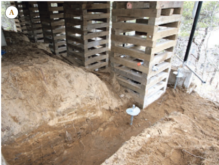
Figure 3. To set up jacking stations and restore the building to a level condition, the crew shoveled out a level base behind the failed grade beam and stacked cribbing under the floor joists (A), leaving just enough room for helical piers (B). Note the steel chain cast into the original grade beam, which was tied back to the foundation in a failed attempt to stabilize the faulty construction.
