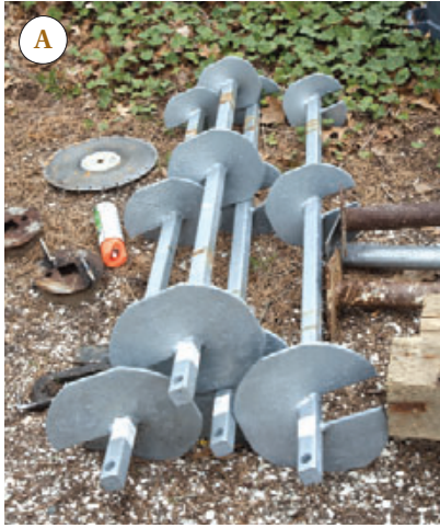
Figure 2. Because of the steep slope and difficult access, the helical piers (A) and extension shafts (B) were driven using a custom-made steel frame to support the auger head (C). An excavator parked at the top of the hill provided hydraulic power (D).
