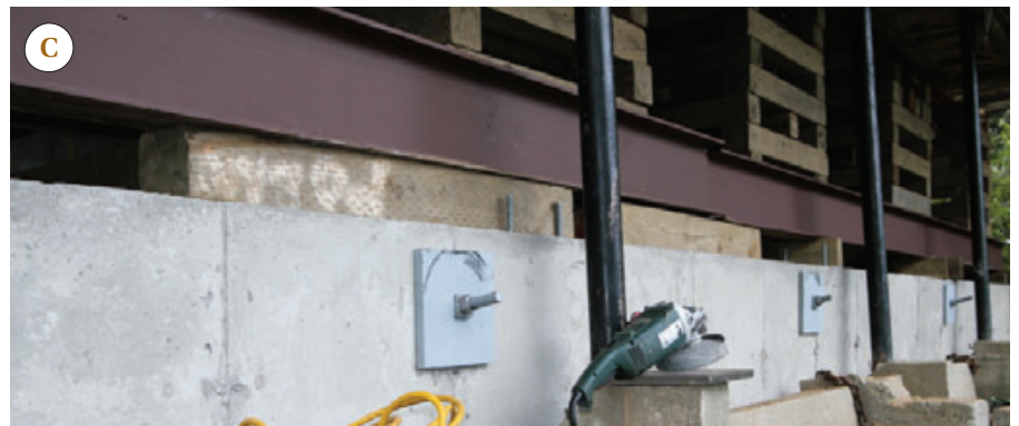
Figure 7. Galvanized connecting rods (A) attached to the angled tie-back piers are run through 4-inch-diameter PVC knockouts (B). Three-quarter-inch-thick steel plates on the outside of the grade beam capture the ends (C). Note the two steel I-beams sitting on top of the grade beam, ready to be welded together to form one long support.
