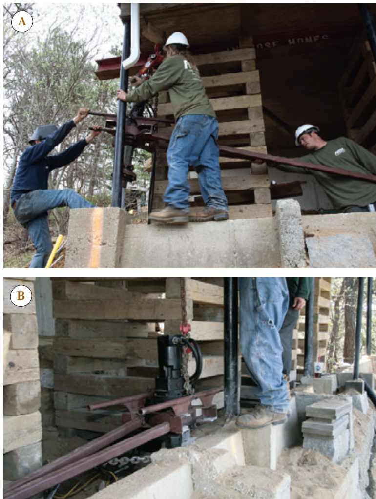
Figure 5. As the required driving force increased (A), a drag bar attached to the auger frame helped counter the reverse torque (B). Space between the cribbing stacks was too tight to use the drag bar; there, the crew struggled to brace the frame against the cribbing without toppling the stacks (C).
