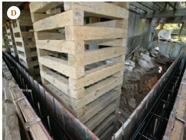
Figure 6. Heavy steel bearing plates welded to the tops of the piers support a beefy rebar cage, which has been spot-welded to the plates (A). Tube forms surround the upper ends of the piers, to encase them in concrete (B). After the last welds are made (C), the grade beam is ready to be poured (D).
