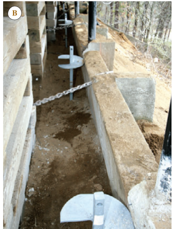
Figure 3. To set up jacking stations and restore the building to a level condition, the crew shoveled out a level base behind the failed grade beam and stacked cribbing under the floor joists (A), leaving just enough room for helical piers (B). Note the steel chain cast into the original grade beam, which was tied back to the foundation in a failed attempt to stabilize the faulty construction.
