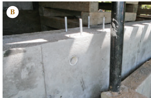
Figure 7. Galvanized connecting rods (A) attached to the angled tie-back piers are run through 4-inch-diameter PVC knockouts (B). Three-quarter-inch-thick steel plates on the outside of the grade beam capture the ends (C). Note the two steel I-beams sitting on top of the grade beam, ready to be welded together to form one long support.
