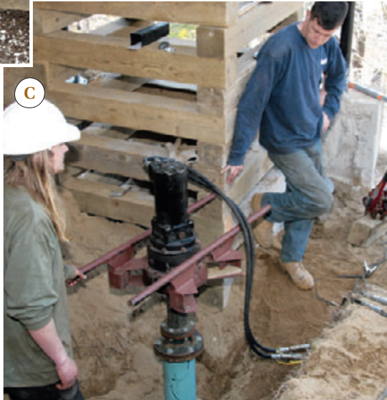
Figure 2. Because of the steep slope and difficult access, the helical piers (A) and extension shafts (B) were driven using a custom-made steel frame to support the auger head (C). An excavator parked at the top of the hill provided hydraulic power (D).
