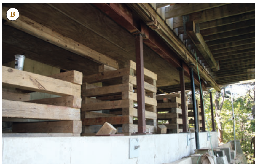
Figure 8. With the building jacked to its final level position, the steel columns were cut to finish height with a portable band saw (A). The steel I-beam was then jacked into place and welded to the tops of the columns (B). Diagonal 4x6 braces anchored atop the grade beam stiffen the cantilevered deck above (C).
