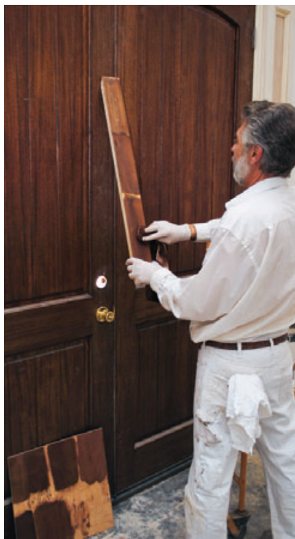
Figure 1. The author prepared sample boards of poplar and birch plywood, the materials used to build the entry trim (far left), then blended different stain colors together to find the combination that would most closely match the color of the stained and seal-coated mahogany entry doors (left).
