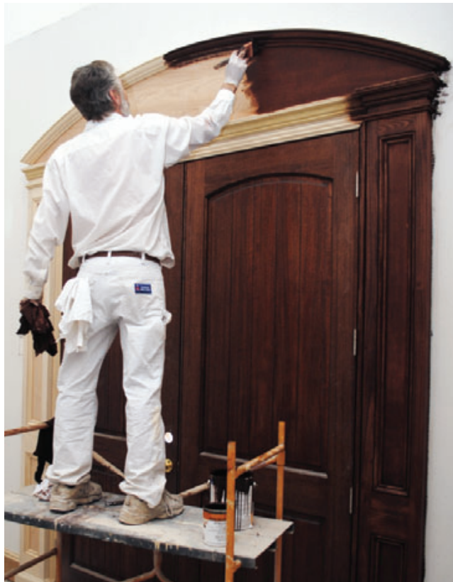
Figure 2. The author brushes the oil-based stain onto each section of trim (left), then wipes it off with a rag to remove the excess and even out the finish (above). After the stain has dried overnight, the trim will receive two coats of fast-drying vinyl sanding sealer.
