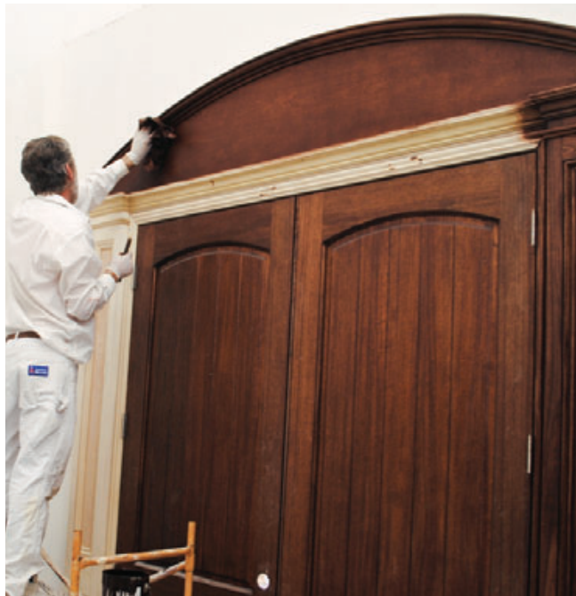
Figure 2. The author brushes the oil-based stain onto each section of trim (left), then wipes it off with a rag to remove the excess and even out the finish (above). After the stain has dried overnight, the trim will receive two coats of fast-drying vinyl sanding sealer.
