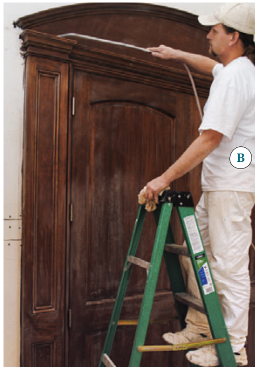
Figure 3. Before the sealed doors and trim can be top-coated, they must be lightly sanded again, typically with fine-grit sanding sponges or 220-grit sandpaper (A). Compressed air is handy for removing sanding dust from cracks (B), but the trim must also be wiped down with a rag dipped in mineral spirits. Then three to four coats of CAB acrylic lacquer are sprayed onto the entire assembly, with a light sanding between coats (C, D).
