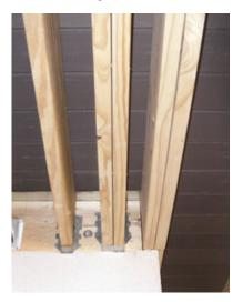
The additional loads the double joist in this photo carries are not assumed in the engineering behind the IRC's new ledger bolting table, so this common connection is now prohibited without further engineering.
