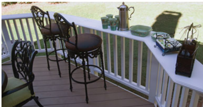
Figure 8. Cap the top of a railing with a PVC board and you have an eye-catching bar top.
