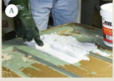
Removing paint with the Peel Away system is a multistep process. First you coat the surface with a thick layer of paste (A), then you cover the paste with paper sheeting and wait for the chemical process to loosen the paint. After 12 to 24 hours, you peel the paint and paper off the surface and dump the whole mess in the trash (B). Last, you wipe down with water and neutralize the chemical using a vinegar solution (C).
