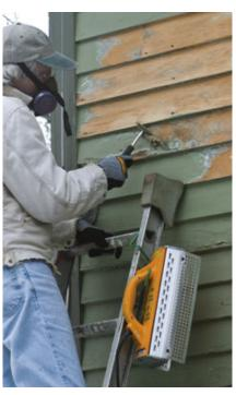
The Speedheater has a multisided profile scraper that allows it to remove paint from moldings (left) as well as flat stock. Unlike high-speed rotary tools that require two hands to operate, it can be used safely on an extension ladder (right).
