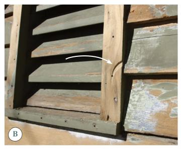
The Paint Shaver's triangular blades (A) can remove unwanted paint from the faces and butts of clapboards at the same time. But in the hands of an inexperienced operator, this powerful tool can easily damage the substrate (B), so it's a good idea to practice on an inconspicuous area. Also, even though the Paint Shaver excels at stripping wide, flat surfaces, it leaves a significant swath of untouched paint in the corners (C) that must be removed by other means.
