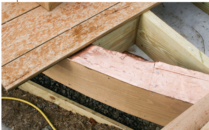
Figure 4. Copper flashing keeps water from collecting in rot-prone areas, such as between double joists.
