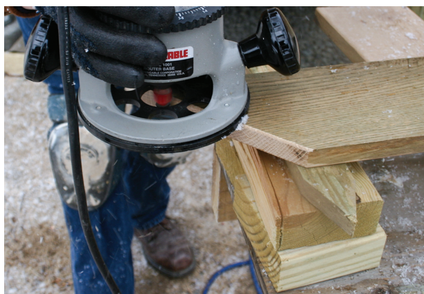
Figure 5. Rounding over the bottom of the cut ends of decking minimizes the amount of end grain in contact with water that puddles on the joists.
