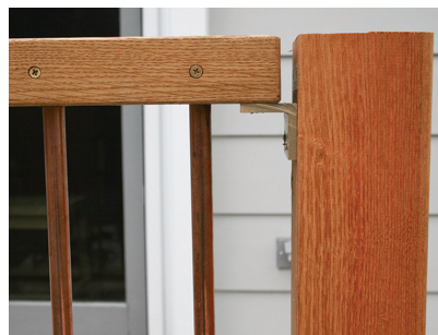
Figure 9. Bronze angle supports the railing and provides an air gap to foster drying at a vulnerable joint.
