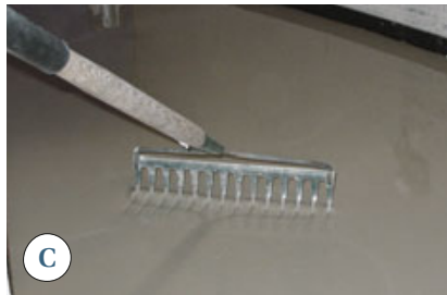
Figure 7. Starting with the low spots, all of the buckets of SLU are poured onto the floor (A). To move material around, the crew uses a flat trowel-like spreading tool (B), a standard garden rake (C), and a gauge rake with adjustable wire sleds (D).
