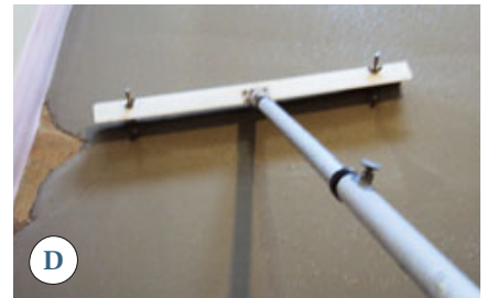
Figure 7. Starting with the low spots, all of the buckets of SLU are poured onto the floor (A). To move material around, the crew uses a flat trowel-like spreading tool (B), a standard garden rake (C), and a gauge rake with adjustable wire sleds (D).
