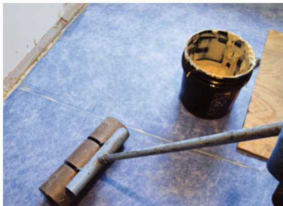
Figure 8. To install this sheet-style antifracture membrane, the crew spreads adhesive with a notched trowel (left), then beds the membrane — already cut to fit — with a roller (above). Once the adhesive has been cleaned up, the floor is ready for tile.
