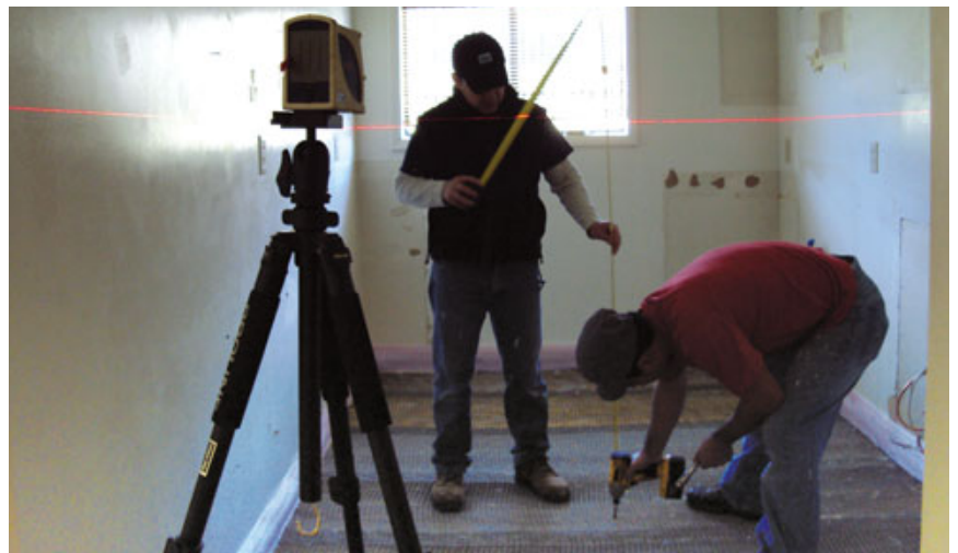
Figure 4. Measuring down from the laser's benchmark elevation, workers drive screws into the floor to identify low spots and mark the final height of the slab.
