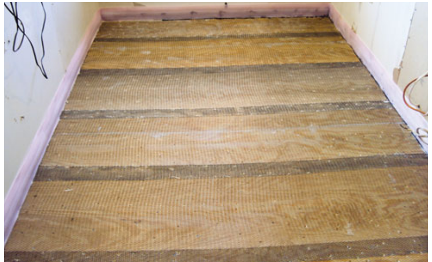
Figure 3. Expanded metal lath is needed over wood subfloors to reinforce the SLU.
