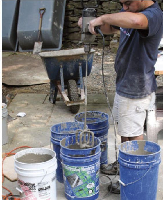
Figure 6. An exact amount of water is dumped into the bucket, and then a bag of powder. Each bag gets its own bucket, and is mixed for two minutes with a 1/2-inch drill equipped with a special mixing paddle.
