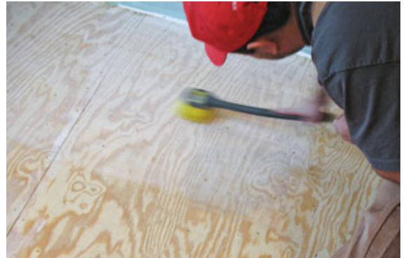
Figure 2. Primer is needed to seal the subfloor. A worker rolls it on (left), then uses a stiff bristle brush to force it into the fibers of the plywood (above).
