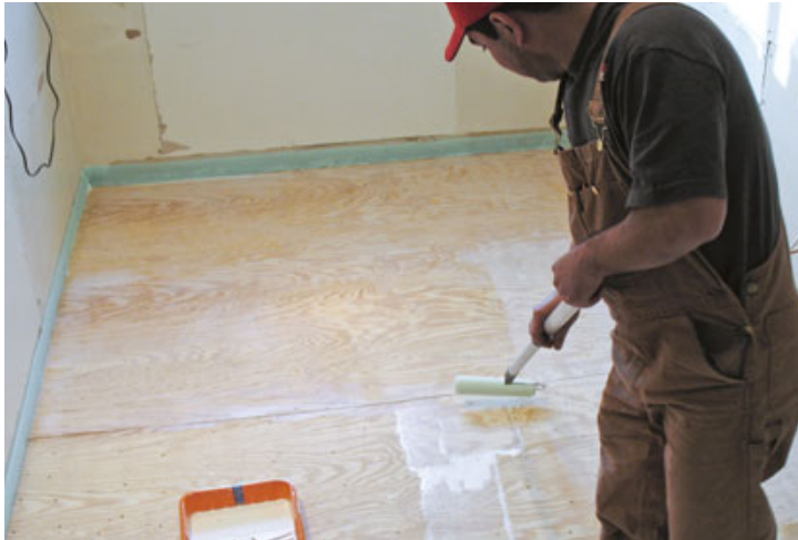
Figure 2. Primer is needed to seal the subfloor. A worker rolls it on (left), then uses a stiff bristle brush to force it into the fibers of the plywood (above).
