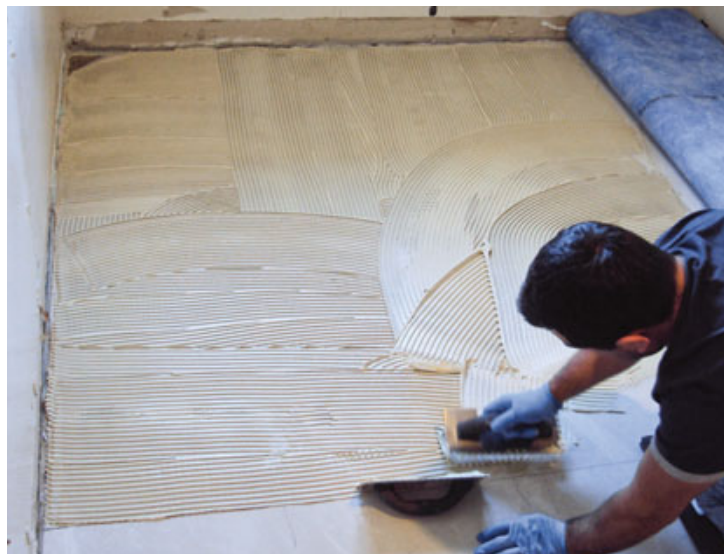
Figure 8. To install this sheet-style antifracture membrane, the crew spreads adhesive with a notched trowel (left), then beds the membrane — already cut to fit — with a roller (above). Once the adhesive has been cleaned up, the floor is ready for tile.
