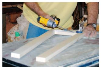
**1.** The tapered center section of the newel is made up of four frame-and-panel assemblies. I transferred the dimensions and angles for the stiles and rails from my full-scale drawing, cut them to width and length from <sup>3</sup>/4-inch poplar, and joined them together with pocket screws and glue.
