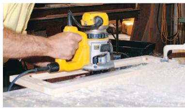
**2.** I then cut a  $^3$ /8-inch rabbet around the inside of each frame with a router to accommodate the plywood panels, which I would make from readily available  $^3$ /4-inch birch plywood.
