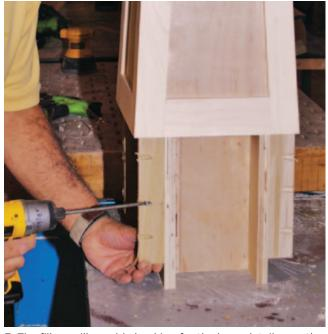
**5.** The fillers will provide backing for the base detail once the newel post is in place, and are positioned so that the base will align with the bottom of the tapered section above.
