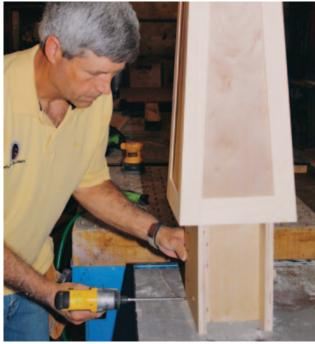
**4.** At the bottom, before nailing off the base of the tapered panels, I built out the column with plywood fillers.
