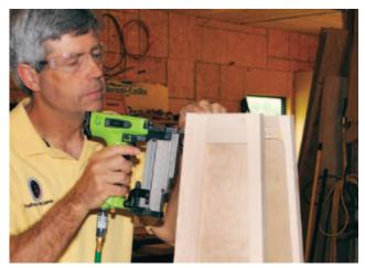
**1.** I glued the four frames together, pinning them to each other with my 23-gauge headless nailer to hold the assembly in place while I set up my clamps.
