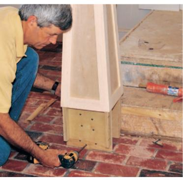
**2.** After a dry fit, I covered the blocking with plenty of construction adhesive and slid the post into place, shimming it plumb and then fastening it to the blocking with long structural screws driven in from three sides.
