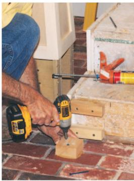
**1.** Before setting the post, I marked the location of the center of the handrail on the landing, then lined up the center of the post with these marks. This helped me locate the blocking needed on the floor and riser for mounting the post.
