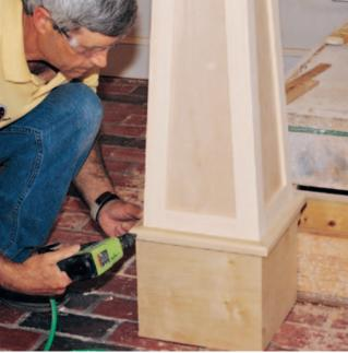
**3.** Finally, I finished the post with a  $9^{1/2}$ -inchwide plywood base, mitering the corners and adding a chamfered cap to hide the joint.
