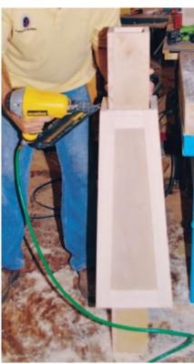
**2.** After flush-sanding the joints on the two panel assemblies, I slid them over the column and nailed them in place, starting with the tapered section.
