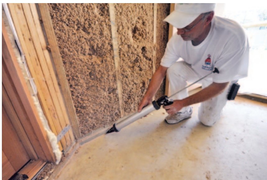
Figure 7. The 2x4 framing adjacent to the doorway (top) has been sprayed with a thin layer of closed-cell foam, which will later be covered with a thicker layer of spray cellulose, already visible on the taller wall at right in the photo. Note how the ceiling above the doorway has been insulated with open-cell foam. Cracks between the slab and bottom plates are sealed with flexible caulk (above); to prevent interference with the drywall and trim, caulk at framing members is immediately tooled flat (right).
