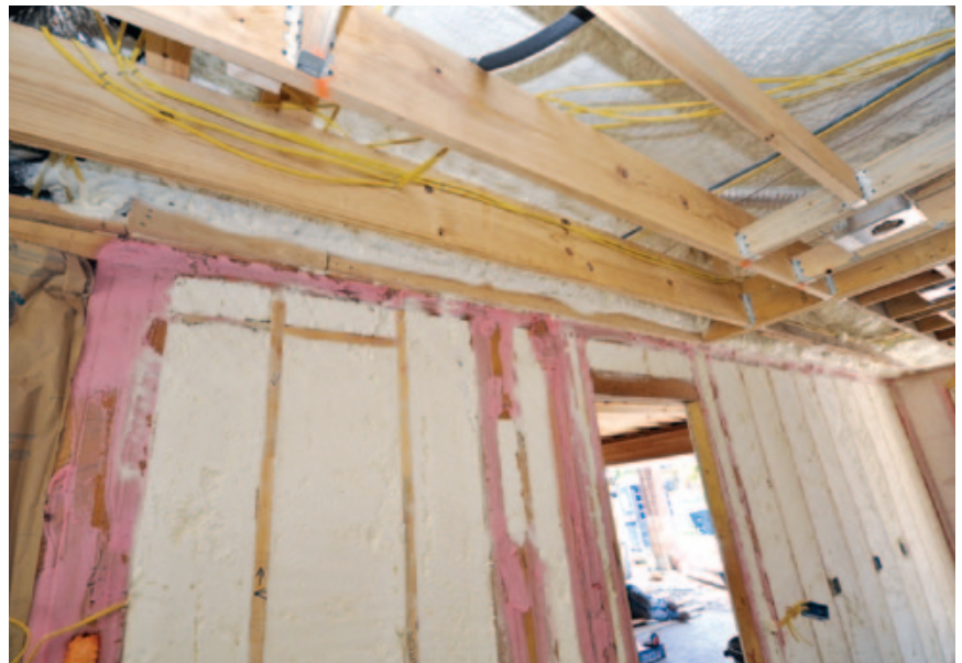
Figure 6. Potential leak points in the framing of this partition between a living space and garage were sealed with sprayable caulk before the foam sub sprayed the cavities and overhead roof deck. Ductwork will be installed in the conditioned space between the roof deck and ceiling, which should improve the performance of the home's air conditioning and heating.
