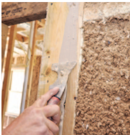
Figure 7. The 2x4 framing adjacent to the doorway (top) has been sprayed with a thin layer of closed-cell foam, which will later be covered with a thicker layer of spray cellulose, already visible on the taller wall at right in the photo. Note how the ceiling above the doorway has been insulated with open-cell foam. Cracks between the slab and bottom plates are sealed with flexible caulk (above); to prevent interference with the drywall and trim, caulk at framing members is immediately tooled flat (right).
