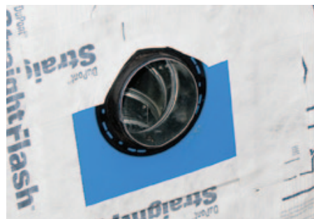
Figure 2. To exclude outdoor air as well as bulk water, this dryer-vent pipe (right) was sealed to the house-wrap with a flexible flashing panel and butyl tape. The same approach was used for a demand water heater's rough-in (above); the gas line is on the right in the photo and the hot and cold water lines are at left.
