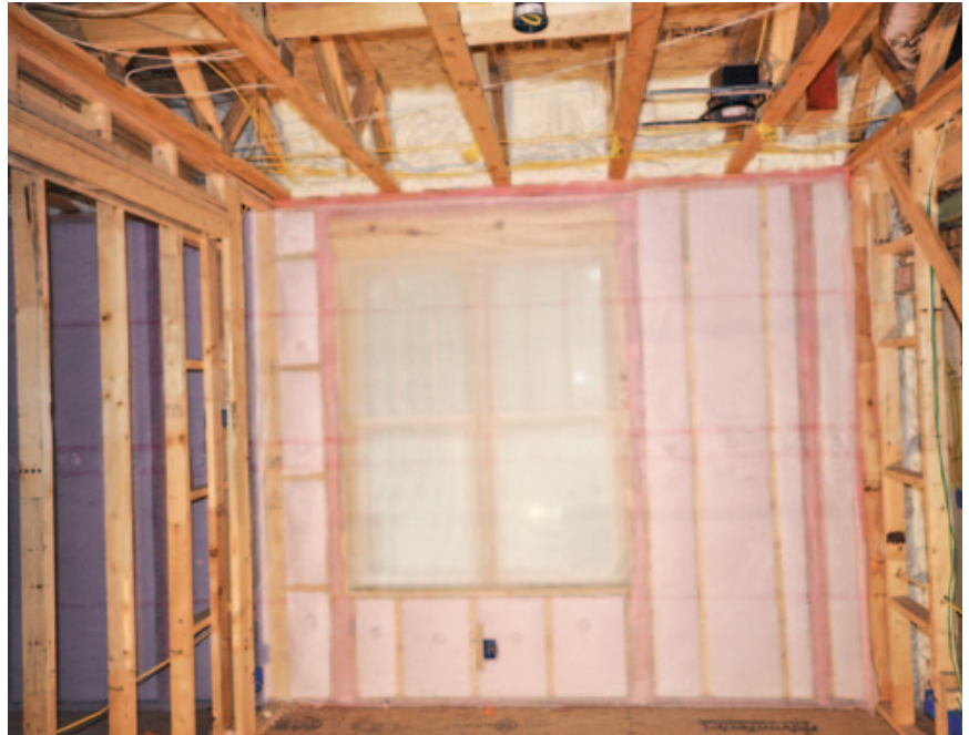
Figure 5. Once the air-sealed framing is covered with staple-up netting, the cavities are filled with blown fiberglass, which the author finds more reliable than batts. According to the manufacturer, the latex sealant is designed for use with either material.
