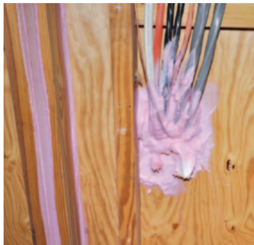
Figure 4. A proprietary spray rig (top) is used to apply flexible latex foam to potential leak points between framing members, between framing and panel edges (above), and at wire penetrations (right).
