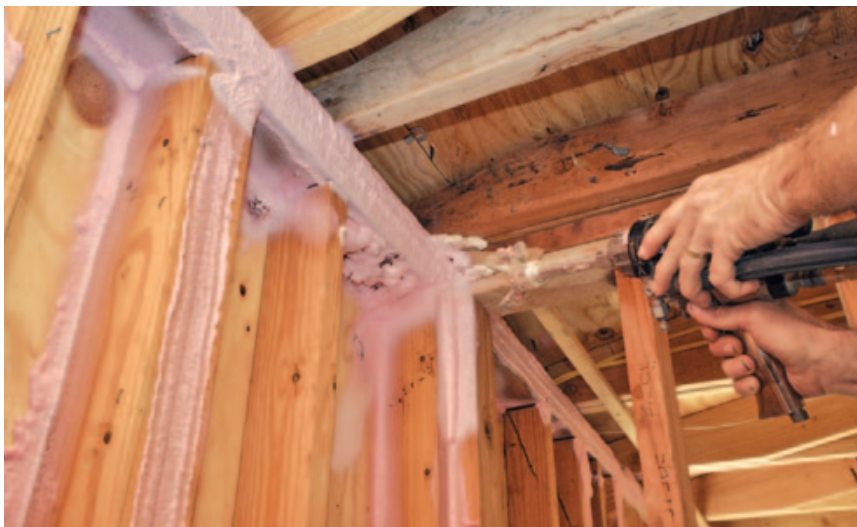
Figure 4. A proprietary spray rig (top) is used to apply flexible latex foam to potential leak points between framing members, between framing and panel edges (above), and at wire penetrations (right).
