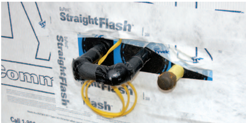
Figure 2. To exclude outdoor air as well as bulk water, this dryer-vent pipe (right) was sealed to the house-wrap with a flexible flashing panel and butyl tape. The same approach was used for a demand water heater's rough-in (above); the gas line is on the right in the photo and the hot and cold water lines are at left.
