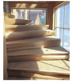
Each individual cedar tread is the full thickness of a riser; the natural curvature of the slab edges provides the code-required nosing. A custom iron railing, not yet installed, will protect the adjacent windows.
