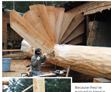
Because they've evolved to bend in the wind, large trees are surprisingly flexible. To eliminate any distortion of the trunk during layout and initial construction of this spiral stair (above), the builders carefully braced the center column in the position it would later assume when vertical (left).
