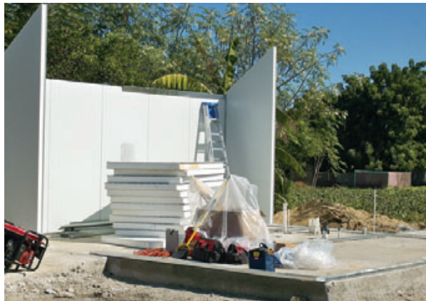
The panels have a T&G friction-fit edge profile and attach to each other and to the galvanized metal base track with screws. The cottage was erected on the existing concrete foundation of a home destroyed by the 2010 earthquake.
