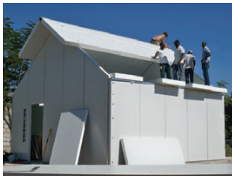
A pair of 8-foot ladders was the only lifting equipment on site. Fortunately, even the 24-foot-long 6-inch roof panels were light enough to be hoisted into place by hand.
