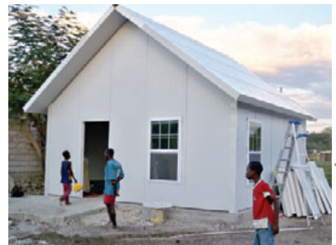
Once the shell was assembled, workers cut out openings and installed the windows and door. The panels' factory-painted coating serves as the interior and exterior finish.
