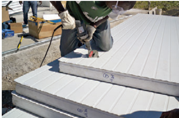
Haitian workers were trained on site to install the steel SIPs, which are made of an EPS core sandwiched between 26-gauge galvanized steel skins. Here, a crew member cuts the gable profile with a Kett panel saw.
