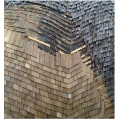
The roofers beveled the edges of opposing shingles that met in the valley bottoms. As each course advanced on a rising curved line out of the valley, the shingle butts were angled to the left or the right as required; the angle decreased from the valleys to the peaks of the lobes. Exposures decreased from the bottom of the structure to the top.
