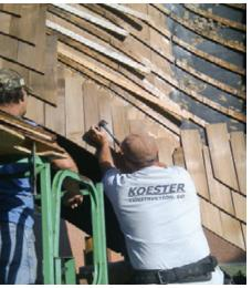
After following the complex layout and cutting all 24,000 replacement shingles with a chop saw on a boom-lift platform, the roofers found the actual hand-nailing to be the easy part. "The goal was to get it right," says contractor Jeff Koester, "not to see how fast we could do it."
