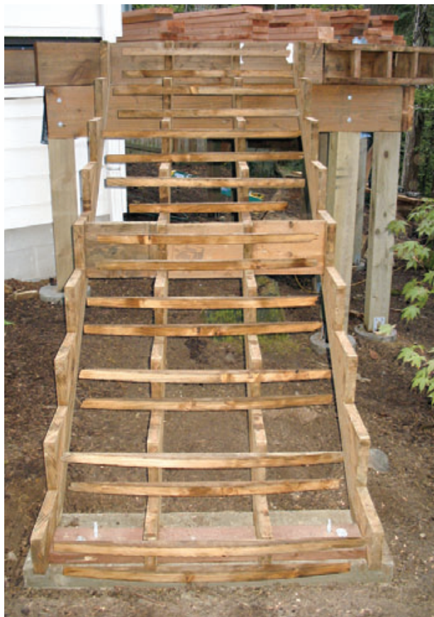
Figure 17. The stair stringers follow the curve of the deck. Blocking cut to that same curve is affixed to the stringers at the top and bottom of each riser.
