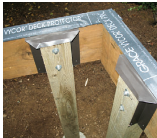
Figure 3. A combination of peel-and-stick membrane and aluminum flashing keeps water out of vulnerable areas.
