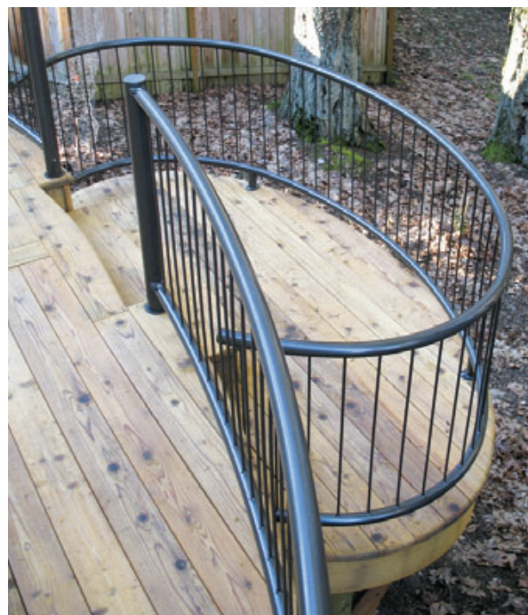
Figure 19. A local metal shop crafted the railings from full-size templates made on site.
