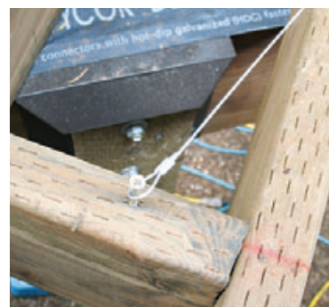
Screws anchor the ends of the cable at the ellipse's foci.
