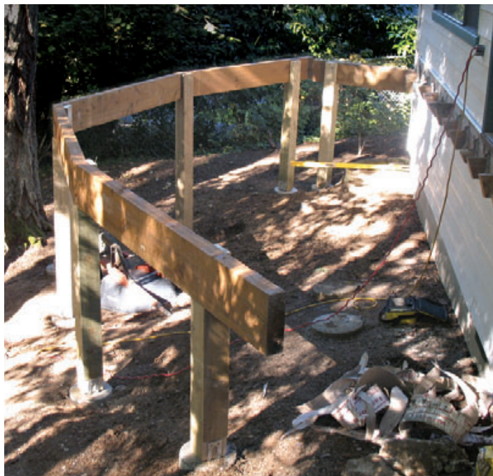
Figure 2. Notched posts supporting beams are a familiar detail throughout the country, but the solid 4x10 beams used here aren't often seen in eastern states. The posts and beams differ in color because they were treated with different preservatives.
