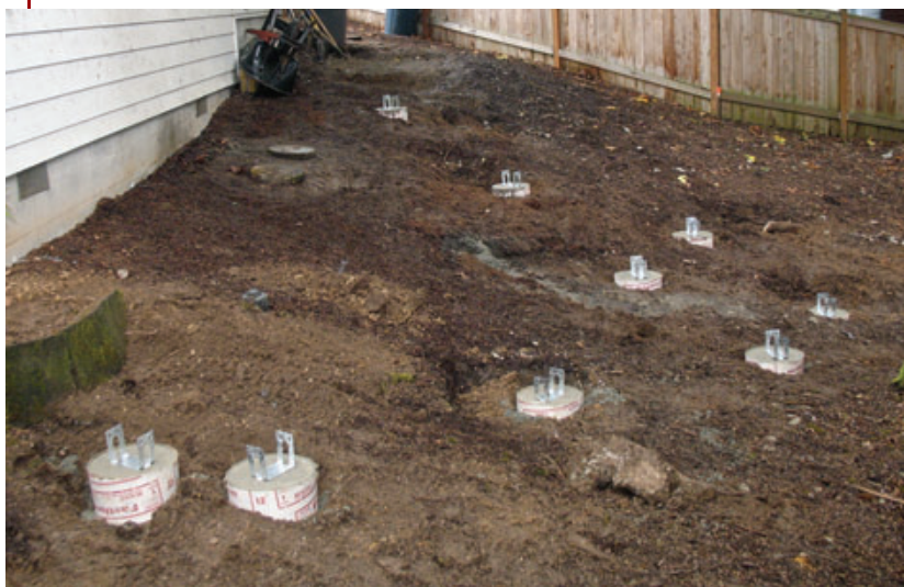
Figure 1. The footings were located to provide a maximum two-foot joist overhang.
