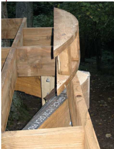
Figure 5. An assembly of blocking and 2x10s on the flat creates the substructure to support the decking at the ends of the ellipse's major axis.
