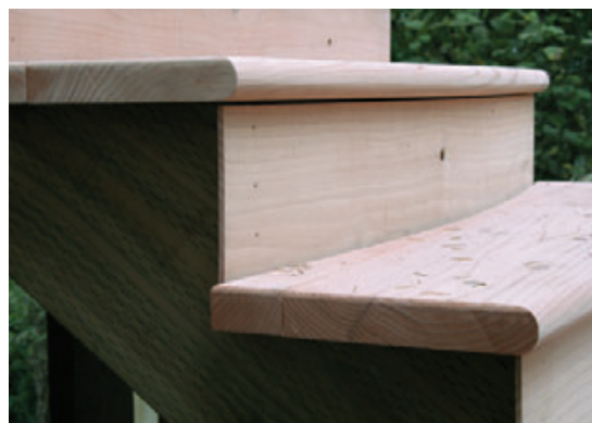
Figure 18. The risers are made from the same material as the fascia. The treads are 2x12s whose fronts are cut to the curve of the ellipse. The offcuts were then fastened to the back of each tread to fit it to the curved riser behind.
