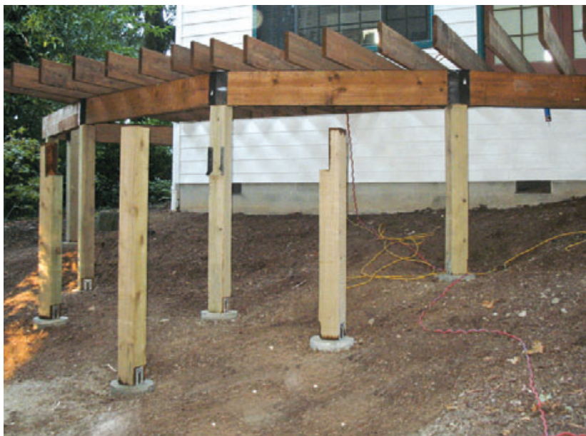
Figure 4. The joists were laid out on 16-inch centers. Their lengths were allowed to run wild; later they would be cut to fit the perimeter of the ellipse.
