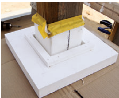
Figure 7. Installation began with the caps (far left) and bases (left) of the structural post surrounds; small cleats attached just inside the column sides provide alignment and backing. The clamping procedure on site was just like that in the shop, except in a vertical position (below left). The purely decorative columns were fitted together — cap, column, base — then slid into place under the beam; here (below), after securing the cap, the author screws the side of the column to the alignment block inside.
