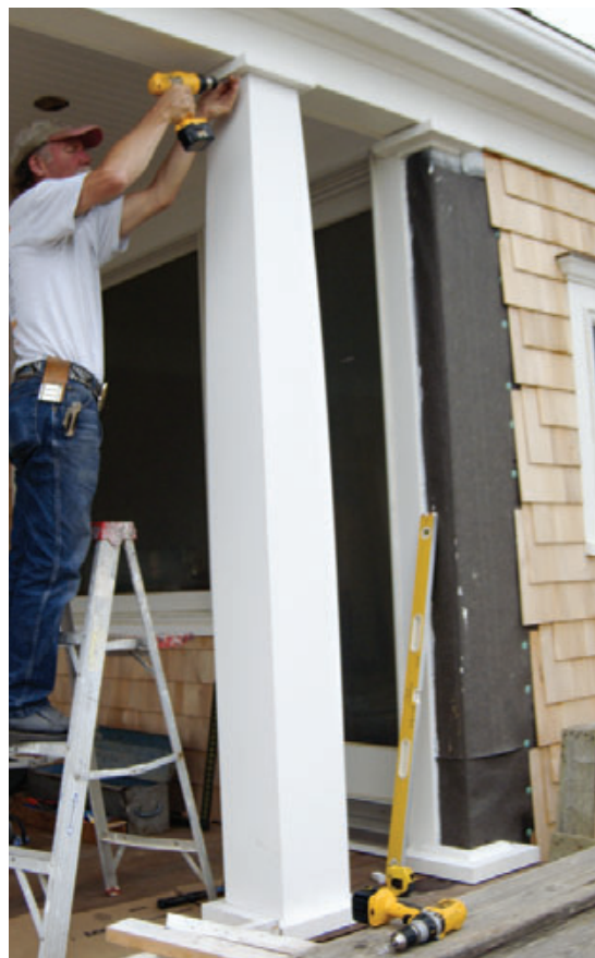
Figure 7. Installation began with the caps (far left) and bases (left) of the structural post surrounds; small cleats attached just inside the column sides provide alignment and backing. The clamping procedure on site was just like that in the shop, except in a vertical position (below left). The purely decorative columns were fitted together — cap, column, base — then slid into place under the beam; here (below), after securing the cap, the author screws the side of the column to the alignment block inside.
