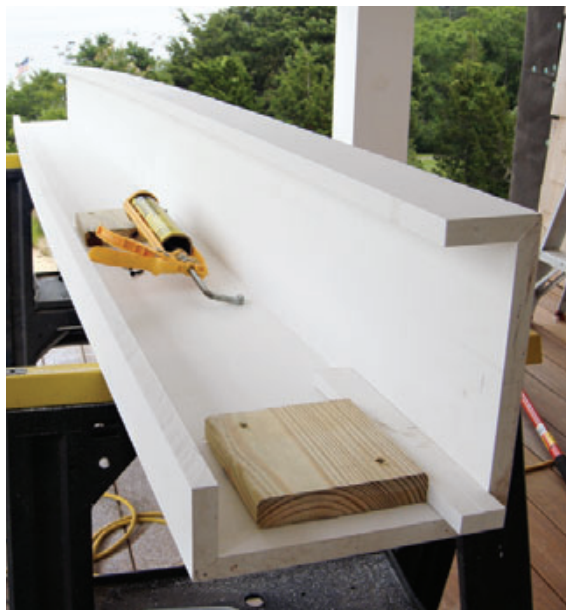
Figure 8. The shingles were held back for installation of the pilasters, which had to be scribed on two sides to the house corners (left). The authors first roughed the scribe cut with a circular saw (above), then installed blocks to catch the handrail and finished the scribing in place.
