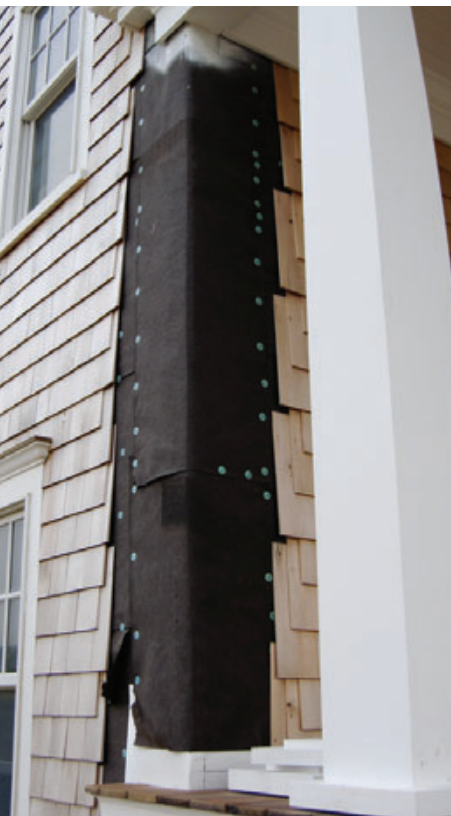
Figure 8. The shingles were held back for installation of the pilasters, which had to be scribed on two sides to the house corners (left). The authors first roughed the scribe cut with a circular saw (above), then installed blocks to catch the handrail and finished the scribing in place.
