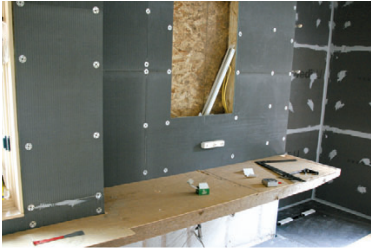
Figure 5. The half-inch-thick Wedi wall panels are installed with special washer-headed fasteners (left). To make the assembly watertight, joints are filled with Wedi's polyurethane sealant (above); for wet areas, the manufacturer also recommends fiberglass mesh tape bedded in thinset.
