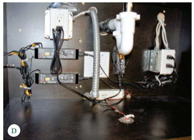
Figure 6. The stained maple vanity cabinet supports an 11-foot-long Kenyan marble countertop with a book-matched front edge (A). The drawers are equipped with LED lighting that turns on automatically when they're opened (B, C). Drivers for the low-voltage LEDs are mounted in the cabinet under the sink (D).
