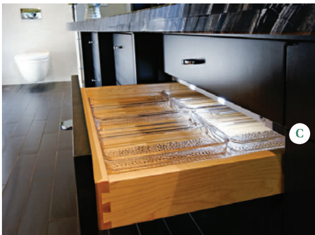
Figure 6. The stained maple vanity cabinet supports an 11-foot-long Kenyan marble countertop with a book-matched front edge (A). The drawers are equipped with LED lighting that turns on automatically when they're opened (B, C). Drivers for the low-voltage LEDs are mounted in the cabinet under the sink (D).
