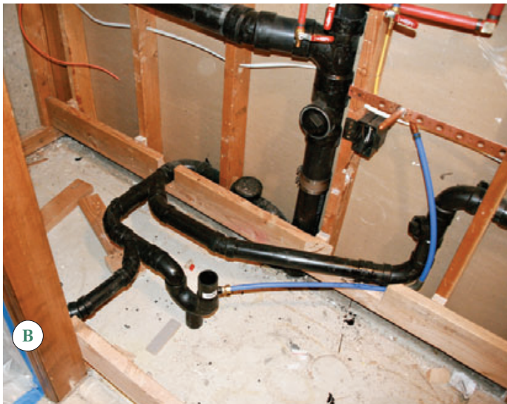
Figure 9. The author converted a basement closet into a small mechanical room with insulated walls and a secondary solid-core door to block noise (A). A new floor framed over the existing slab provides room for drain pipes and a trap primer (B). The subfloor was lined with a galvanized pan fitted with a drain (C). The closet contains a 50-gallon hot-water tank, a small electric boiler for the bathroom's hydronic heating system (D), and the remote shower valve.
