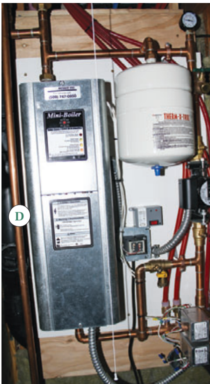
Figure 9. The author converted a basement closet into a small mechanical room with insulated walls and a secondary solid-core door to block noise (A). A new floor framed over the existing slab provides room for drain pipes and a trap primer (B). The subfloor was lined with a galvanized pan fitted with a drain (C). The closet contains a 50-gallon hot-water tank, a small electric boiler for the bathroom's hydronic heating system (D), and the remote shower valve.
