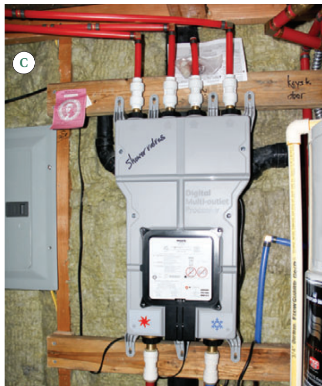
Figure 8. The multihead shower (A) is operated by hand-held remote control (B), so the user can turn it on without getting wet. Water is distributed to the showerheads via a digitally controlled shower valve in the basement (C).
