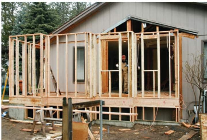
Figure 1. Both the stepped stem wall for the new addition and the old bumpout are visible at left. The author's crew framed the addition walls with engineered studs — which are straighter than sawn studs — to speed wall tile installation (above).
