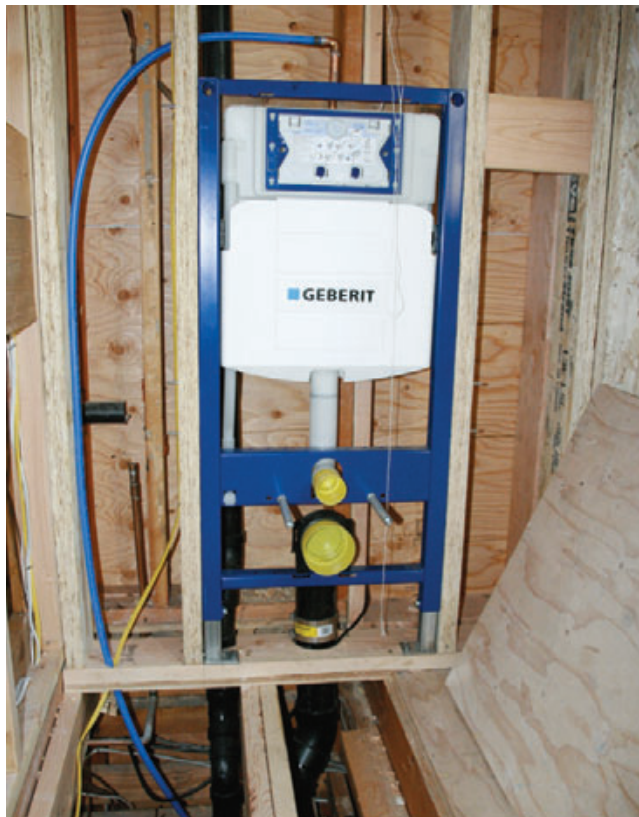
Figure 2. Double-wall framing behind the toilet allowed the waste pipe to be moved out from the foundation wall and made room for extra insulation.
