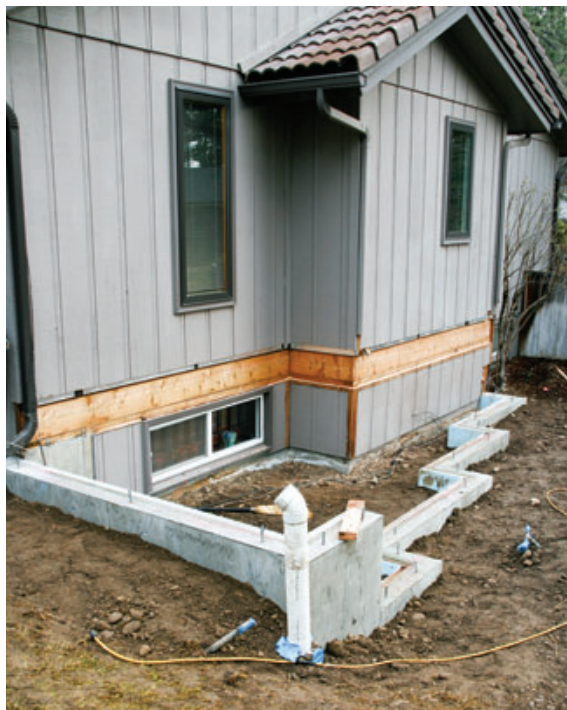
Figure 1. Both the stepped stem wall for the new addition and the old bumpout are visible at left. The author's crew framed the addition walls with engineered studs — which are straighter than sawn studs — to speed wall tile installation (above).
