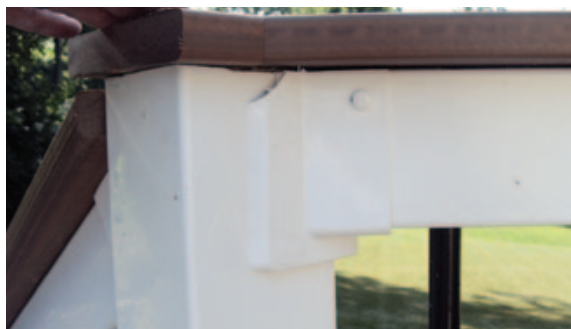
Adding cap rails to standard railings may require field-modifying the brackets.
