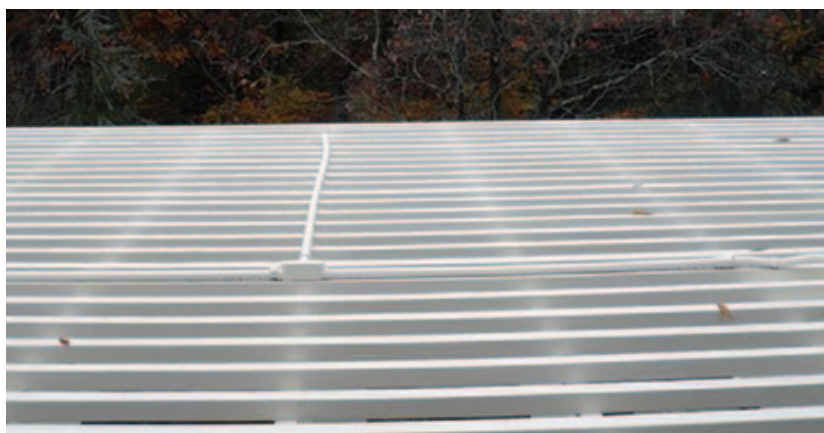
Figure 7. Hiding wiring in an arbor can be a challenge. Running it behind posts and atop the lath are two tricks of the trade.
