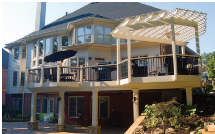
Figure 3. Bolting the posts to the framing provides a great deal of rigidity. With freestanding arbors, more bracing may be needed — in the form of knee braces or, as in the photo, triangular shapes made by the lath, joists, and beams.
