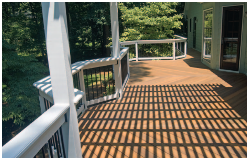
▼ Figure 2. In the middle of the day, most of an arbor's shade comes from the lath. Tightening the spacing provides more shade.
