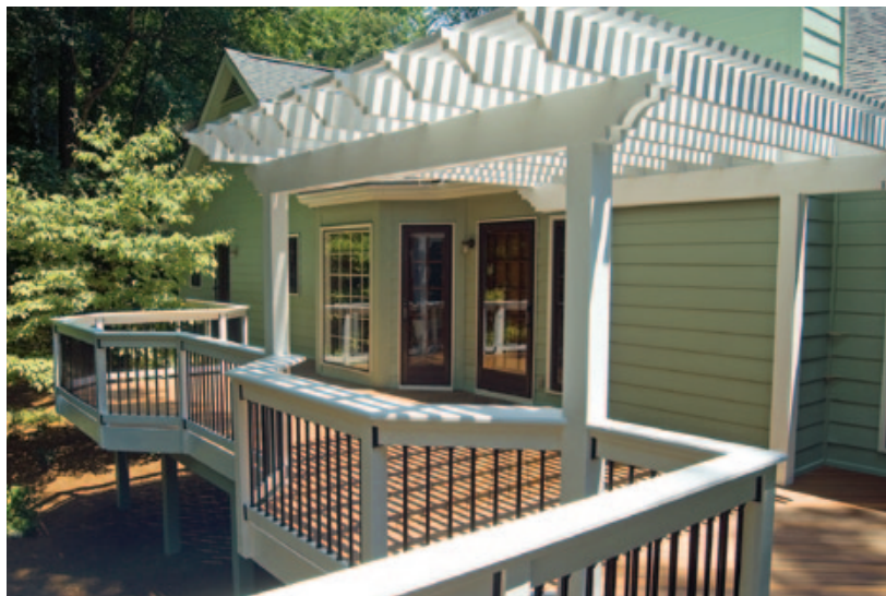
◀ Figure 1. Arbors built from framing lumber create shade and define outdoor rooms. Scroll cuts on the ends of the beams and joists provide interest, and attachment to the house provides rigidity.
