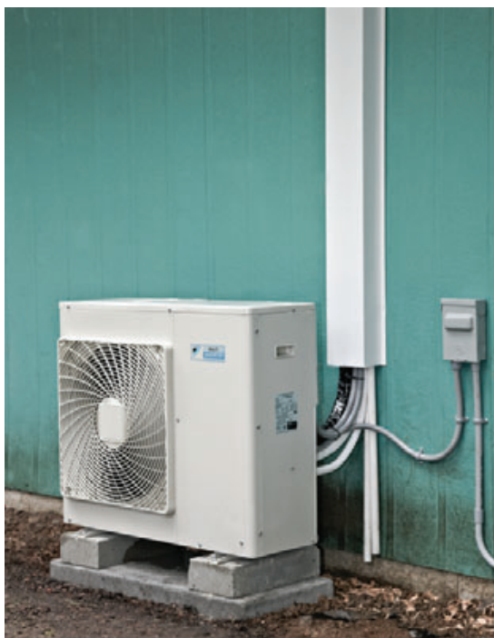
Figure 8. Refrigerant lines and wiring on the exterior wall are protected with a vinyl or sheet-metal cover. Condensate drain tubes are visible at lower right.
