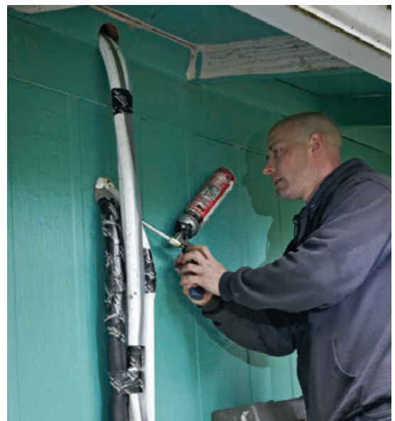
Figure 5. After the mounting bracket of a wall-mounted indoor unit is screwed to the studs (top), the unit itself is hung on the bracket, with the stubs for refrigerant lines, a condensate drain, and an electric line passing through a hole in the exterior wall (center). The 2 9 / 16 -inch hole is later filled with canned closed-cell foam and waterproofed with caulk (above).
