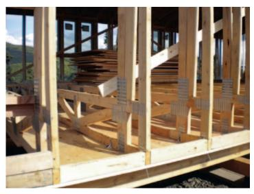
Blocking between trusses took the place of a conventional bottom plate; a  $^3/8$ -inch plywood skin beneath the bottom chords of the open-web floor assemblies served as backing for a thick layer of polyurethane spray foam. An open space between the upper surface of the foam and the subfloor above provided an unobstructed and frostproof plumbing chase.
