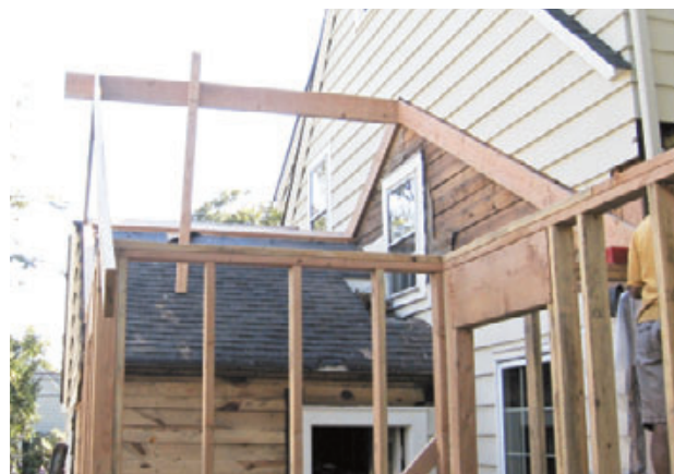
Figure 3. Instead of lowering the new mudroom floor to match the elevation of the old entry into the garage, as called for by the plans (left), the author took advantage of an extension to the garage roof (above) to create headroom above the old garage. This allowed him to raise the entryway and keep the mudroom floor at the same level.
