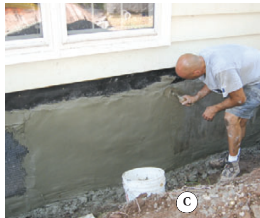
Figure 2. The architect specified a pressure-treated pony wall for resolving a grade problem along the side of the house. The crew exposed the foundation and framing, applied a coat of cold asphalt to the rim-joint area (A), then installed PT sheathing (B). Next, after prepping the wall with 30-pound asphalt felt paper and metal lath, they parged the new and existing walls (C). A second coat of cold asphalt on the below-grade portions of the parged walls (D) — along with drainpipe set in coarse stone wrapped with filter fabric — helps manage water around the foundation (E).
