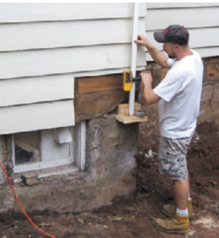
Figure 1. To establish an accurate benchmark elevation for the addition, a carpenter exposes the floor framing in the center of the proposed opening (left). The existing joists were later trimmed or shimmed — and in some cases reinforced with sistered 2x10s — to smooth out the transition into the addition and to prep the kitchen for new wood-strip flooring (below).
