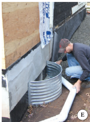
Figure 2. The architect specified a pressure-treated pony wall for resolving a grade problem along the side of the house. The crew exposed the foundation and framing, applied a coat of cold asphalt to the rim-joint area (A), then installed PT sheathing (B). Next, after prepping the wall with 30-pound asphalt felt paper and metal lath, they parged the new and existing walls (C). A second coat of cold asphalt on the below-grade portions of the parged walls (D) — along with drainpipe set in coarse stone wrapped with filter fabric — helps manage water around the foundation (E).
