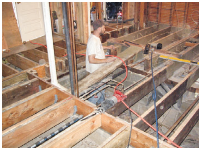
Figure 1. To establish an accurate benchmark elevation for the addition, a carpenter exposes the floor framing in the center of the proposed opening (left). The existing joists were later trimmed or shimmed — and in some cases reinforced with sistered 2x10s — to smooth out the transition into the addition and to prep the kitchen for new wood-strip flooring (below).
