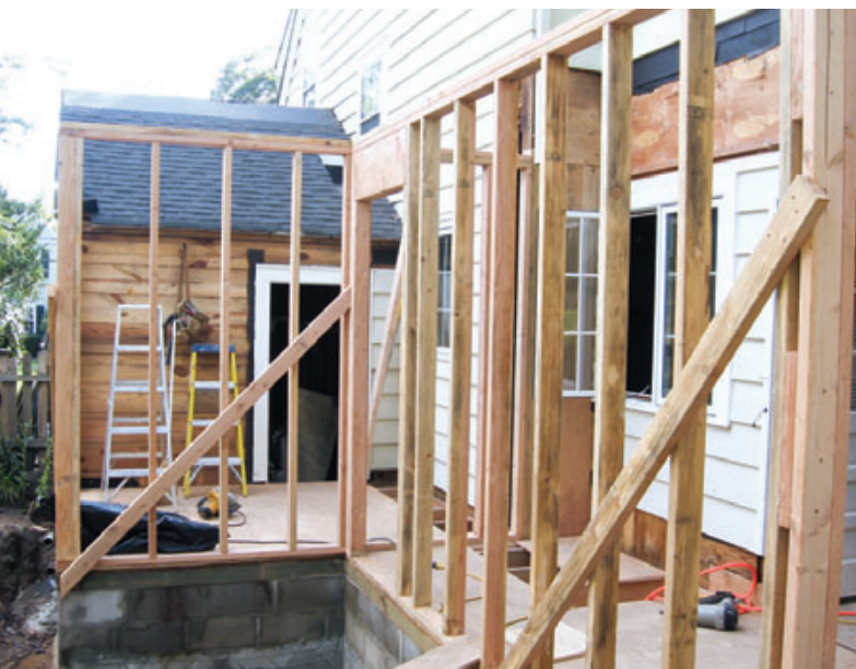
Figure 3. Instead of lowering the new mudroom floor to match the elevation of the old entry into the garage, as called for by the plans (left), the author took advantage of an extension to the garage roof (above) to create headroom above the old garage. This allowed him to raise the entryway and keep the mudroom floor at the same level.
