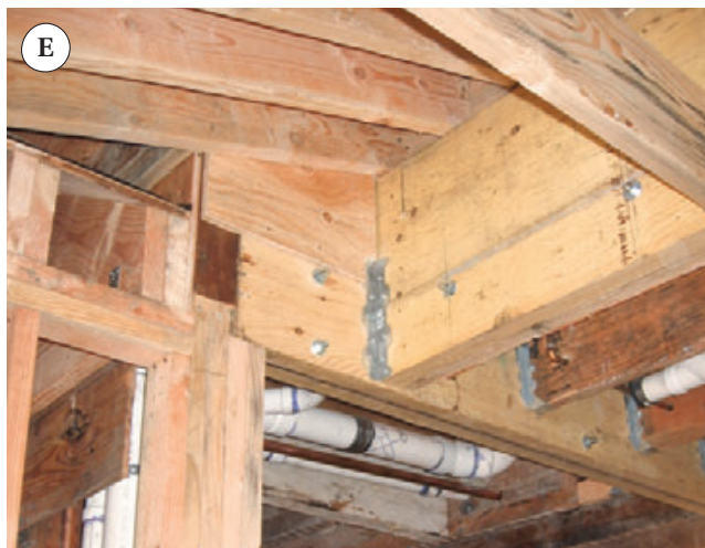
Figure 4. Before opening up the house's rear wall, the crew bolted a pair of 1 3 / 4 -inch by 18-inch LVLs through the exterior sheathing and into the second-story floor framing to support the shed roof of the addition and the second-story framing of the main house (A). Once the house wall was removed (B), they added ceiling joists flush with the existing ones on the other side of the beam. To open up the new eating area, they also replaced an old dropped header with a new fitch beam, first cutting back the joist ends, then slipping it into place (C, D). The two new headers intersect near a support post (E), as indicated in the drawing (facing page).
