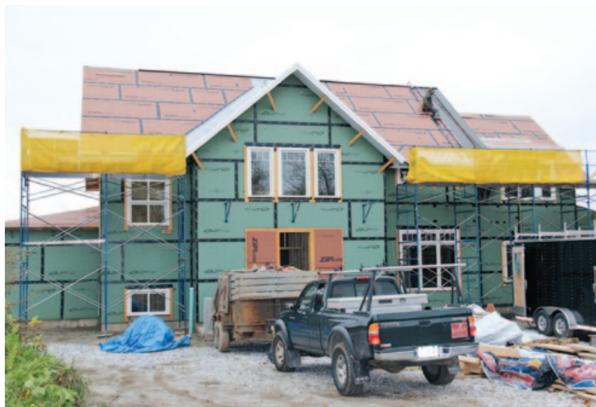
Figure 5. Harnesses may not be needed when there is fully planked staging up to the eaves of a house with guardrails installed as shown. But workers on the cross-gable still need fall protection, because they would be within 6 feet of an unguarded roof edge.
