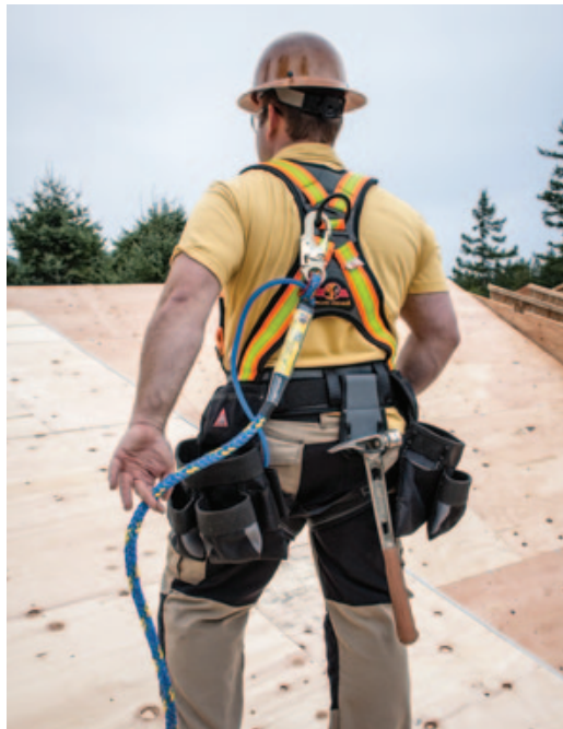
Figure 1. The full body harness at left (superanchor.com) has multiple D-rings, integral tool bags, and a hammer holder, and comes in different sizes. Here it's connected to Super Anchor's X-Line, which combines a 50-foot safety line with a pneumatic air hose. The harness included with the Compliance-in-a-Can kit (right) offers fewer features but is also OSHA-compliant.
