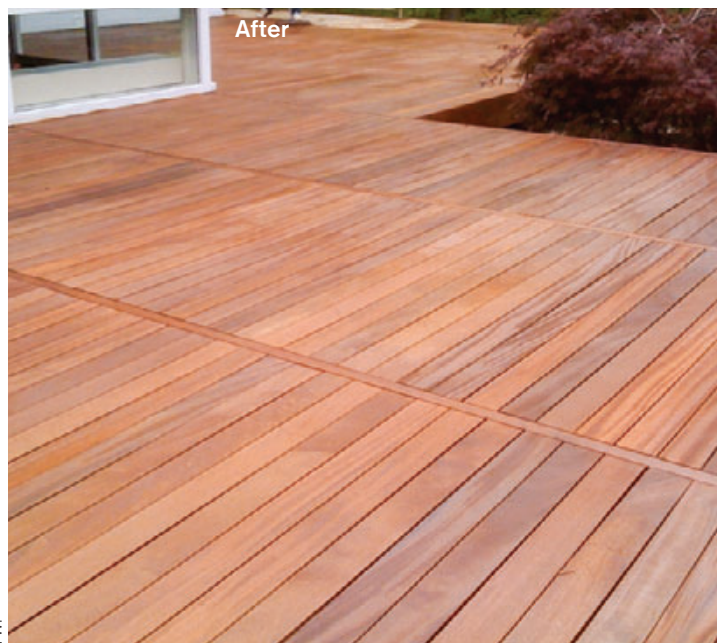
Figure 7. Left unstained, this ipe deck grayed as a natural result of UV exposure (top). Known as photochemical degradation, it's unavoidable unless you use a color-enhanced finish, like toner or stain. A deck brightener was used to remove most of the gray and even out the wood's tone, then a semi-transparent stain brought life back to the wood with a rich color, adding protection from the sun's UV rays (bottom).
