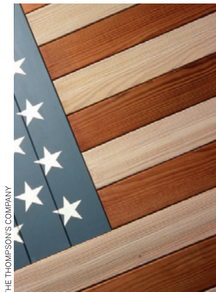
Figure 1. While traditional water-repelling clear finishes allow wood to gray from the sun, colored products block UV-rays for further protection. Toners, like the red shown here, and semi-transparent stains allow grain to show through. Solid stains, like the white and the blue, hide the grain and provide the most protection from UV rays.
