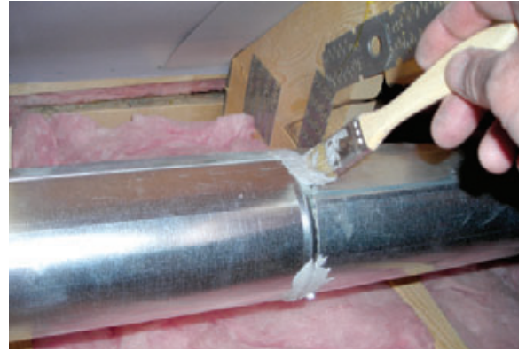
Figure 5. Canned spray foam seals the fan to the dry-wall ceiling (left). Duct mastic seals connections in the pipe (above). Pipe seams were placed up to prevent condensation from leaking out.
