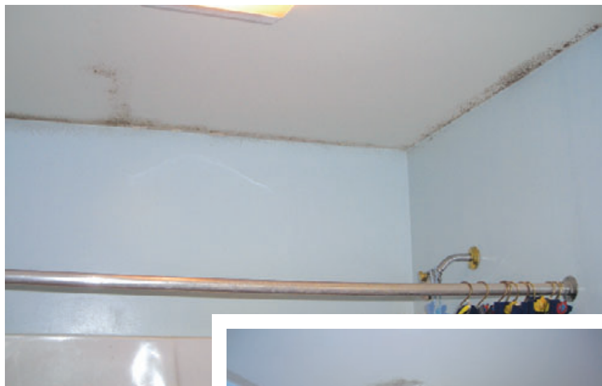
Figure 1. Mold and mildew growing on the bathroom ceilings was all the evidence needed that the ventilation fans were not working effectively. The oblong stain on the ceiling of the shared bath (below) was curious.
