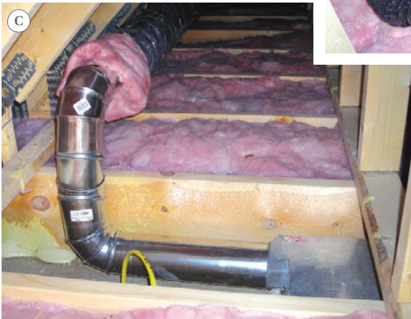
Figure 6. Although insulated plastic flex duct doesn't perform as well as rigid metal duct, it's a handy source for insulation. The author slips the flex duct over the end of the rigid duct (A) and gradually slides it into place as the plastic inner sleeve comes out the trailing end (B). Between the joists around the fan (C), hand-placed cellulose provides excellent coverage (D).
