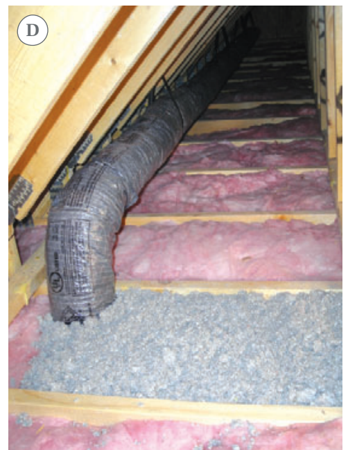
Figure 6. Although insulated plastic flex duct doesn't perform as well as rigid metal duct, it's a handy source for insulation. The author slips the flex duct over the end of the rigid duct (A) and gradually slides it into place as the plastic inner sleeve comes out the trailing end (B). Between the joists around the fan (C), hand-placed cellulose provides excellent coverage (D).
