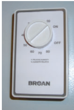
Figure 7. To ensure that lingering moist air is exhausted after a shower, the fan's on/off switch (far left) can be set to turn off at various periods. A humidistat (left) wired in parallel will also turn on the fan when needed.
