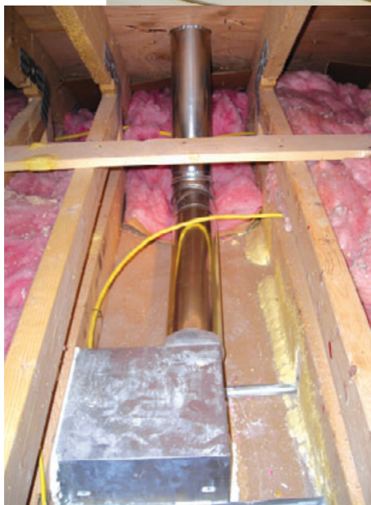
Figure 4. The home's two bath fans originally shared a common rooftop vent termination. To improve performance, the author installed a new gable vent for the shared-bath fan (top), placing the hood under the rake overhang for protection from the weather (above). The master-bath fan was vented to a new roof termination nearby (left).
