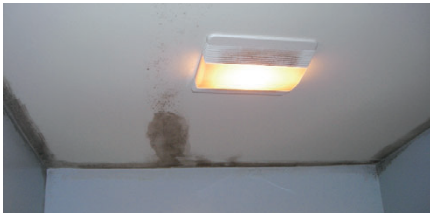
Figure 1. Mold and mildew growing on the bathroom ceilings was all the evidence needed that the ventilation fans were not working effectively. The oblong stain on the ceiling of the shared bath (below) was curious.
