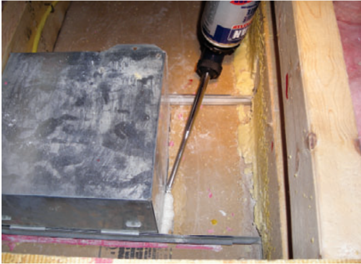
Figure 5. Canned spray foam seals the fan to the dry-wall ceiling (left). Duct mastic seals connections in the pipe (above). Pipe seams were placed up to prevent condensation from leaking out.
