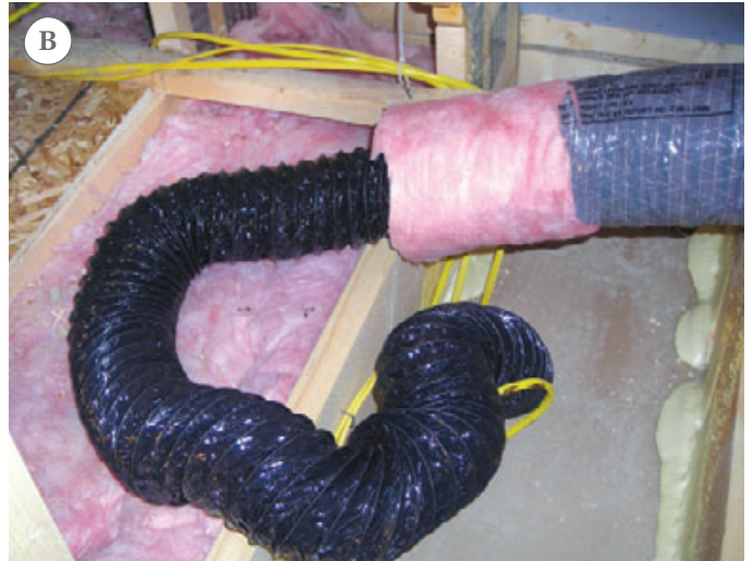
Figure 5. Canned spray foam seals the fan to the dry-wall ceiling (left). Duct mastic seals connections in the pipe (above). Pipe seams were placed up to prevent condensation from leaking out.
