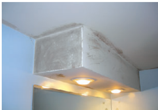
Figure 1. Mold and mildew growing on the bathroom ceilings was all the evidence needed that the ventilation fans were not working effectively. The oblong stain on the ceiling of the shared bath (below) was curious.
