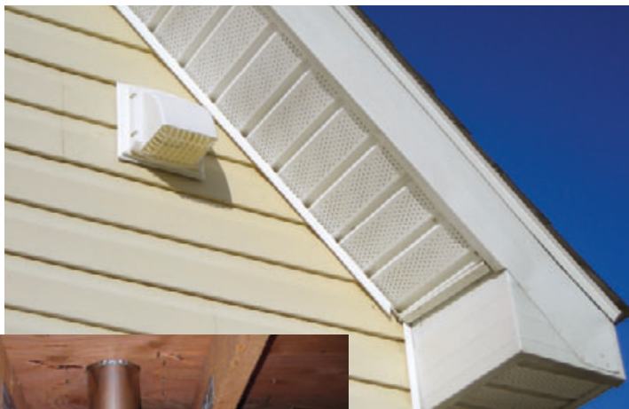
Figure 4. The home's two bath fans originally shared a common rooftop vent termination. To improve performance, the author installed a new gable vent for the shared-bath fan (top), placing the hood under the rake overhang for protection from the weather (above). The master-bath fan was vented to a new roof termination nearby (left).
